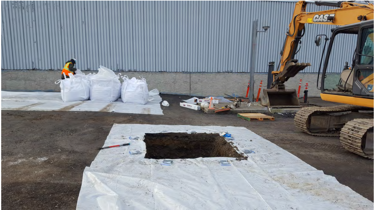
Photo 1: AOC02-005. November 4, 2017 - facing west.
