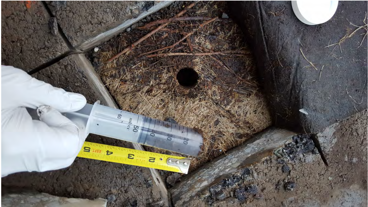
Photo 7: Sod sampling and asphalt removal at AOC08-005. November 3, 2017.
