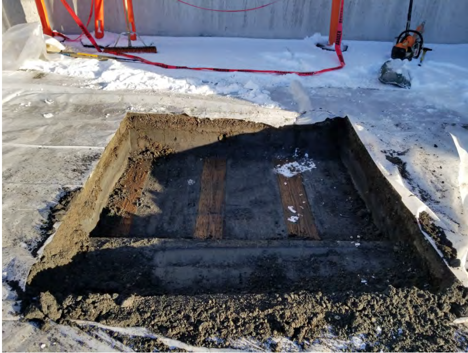
Photo 5: Railroad tracks uncovered during excavation of AOC07-002. November 6, 2017 - facing east.
