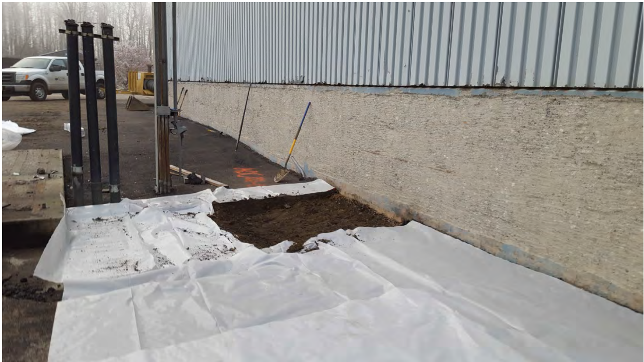
Photo 2: AOC02-008 after sod removal but before excavation. November 4, 2017 - facing south.
