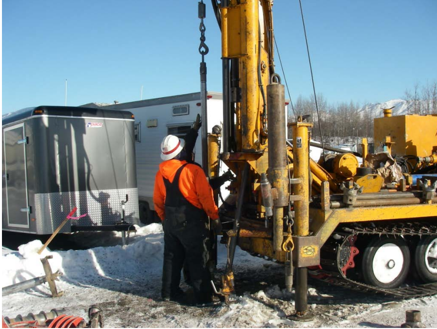
Photograph 3: View to the north of drill rig setting up at TB-10.
