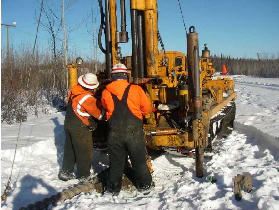
Photograph 1: A view looking north of drilling activities at T-16.
