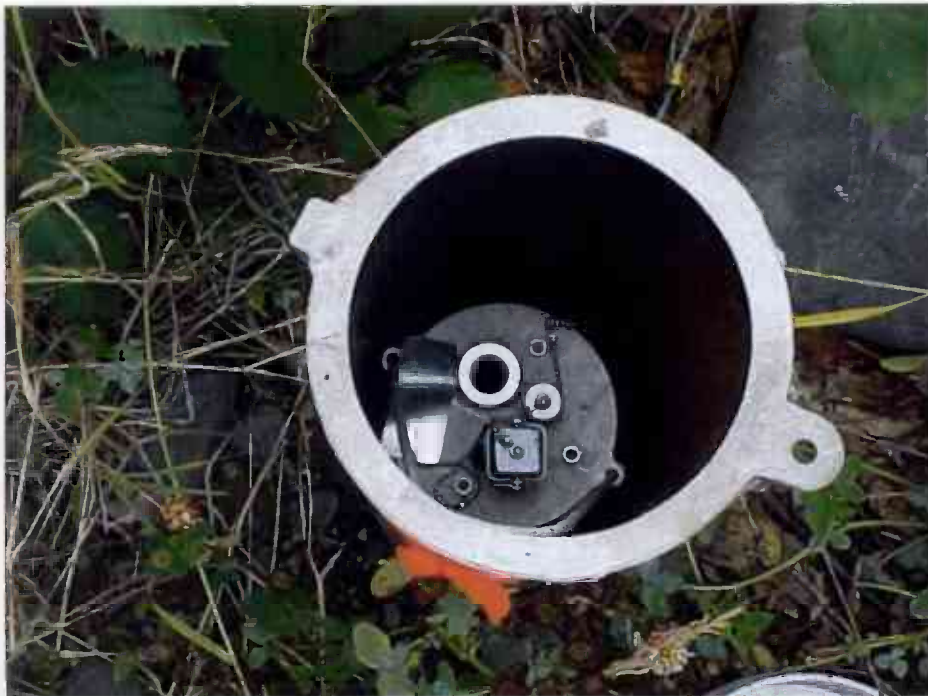
OUB: Poleline Road, Interior View of Monitoring Well AP-4017.
