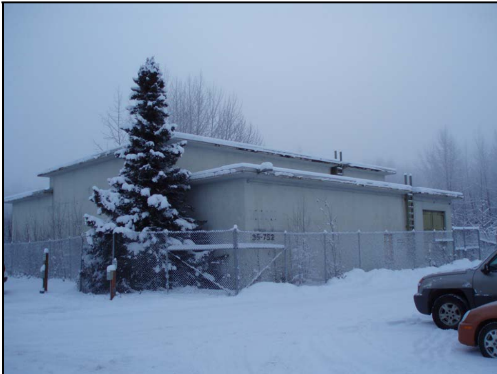
Photograph 9. Security fence around OUE Building 35-752.
