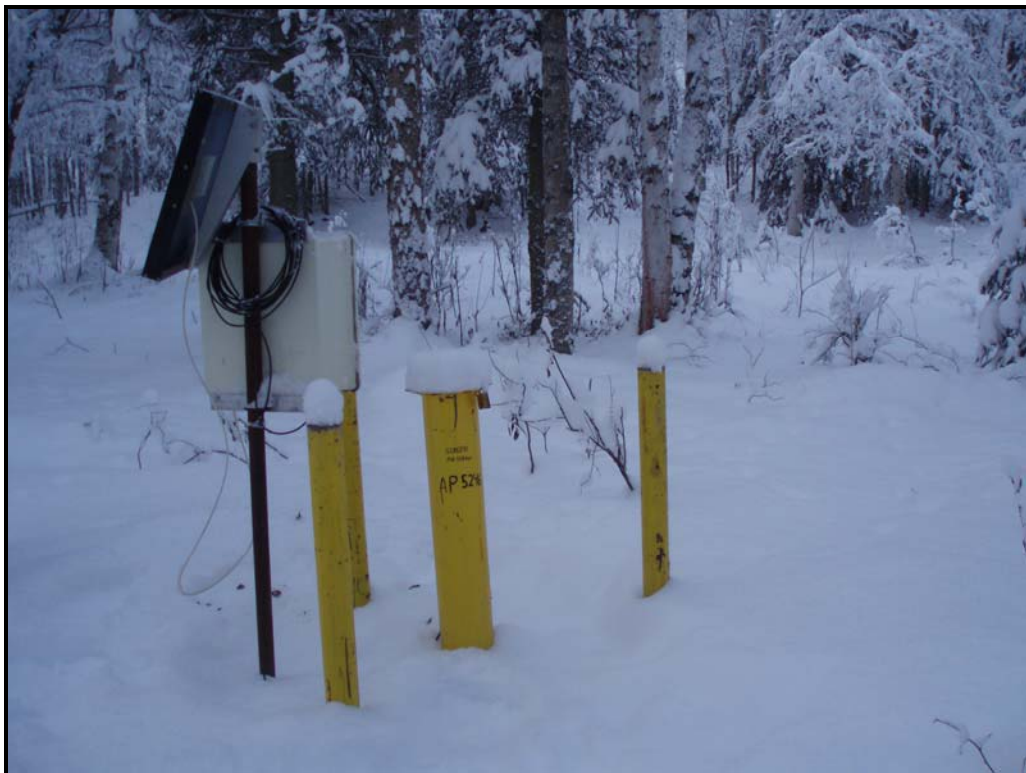
Photograph 4. Monitor well with data logger at OUB Poleline Road site.
