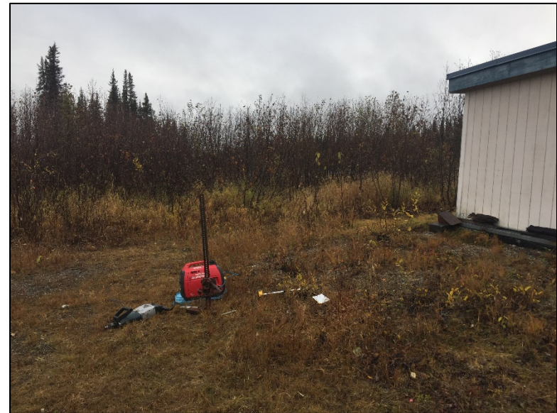
Installing soil boring RSE-9, looking south
