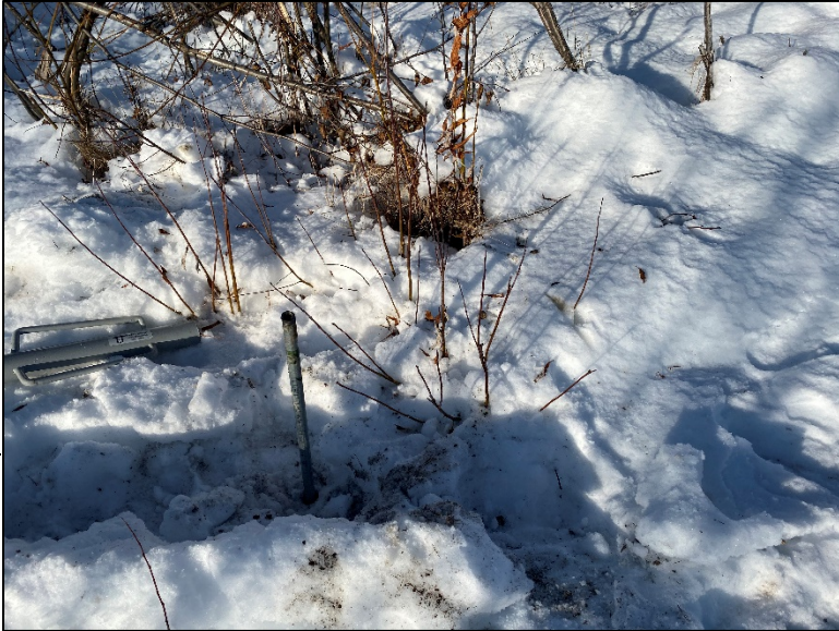
Installing piezo for groundwater sampling at RSE-5, looking southwest
