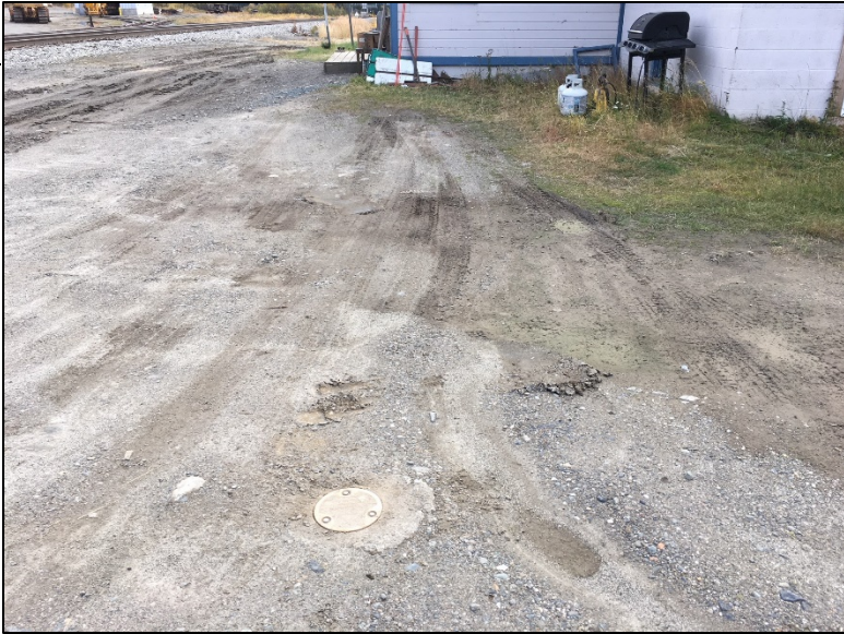
RSE-1, looking north
