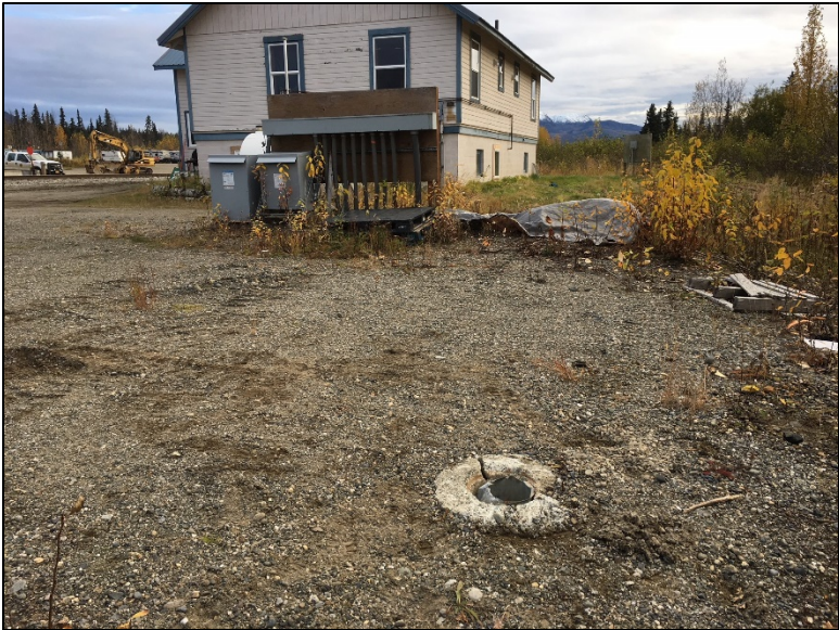
RSE-3, looking northwest
