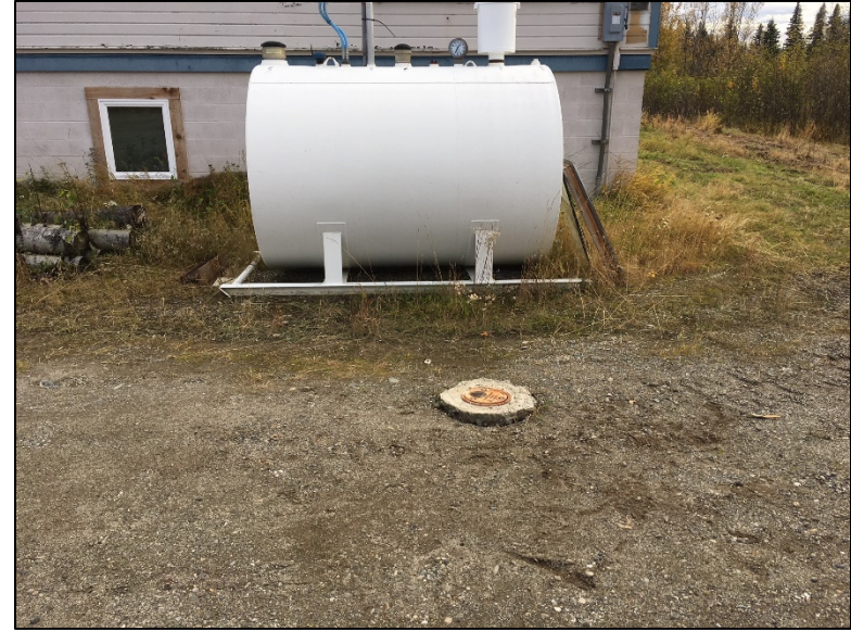
RSE-2, looking north
