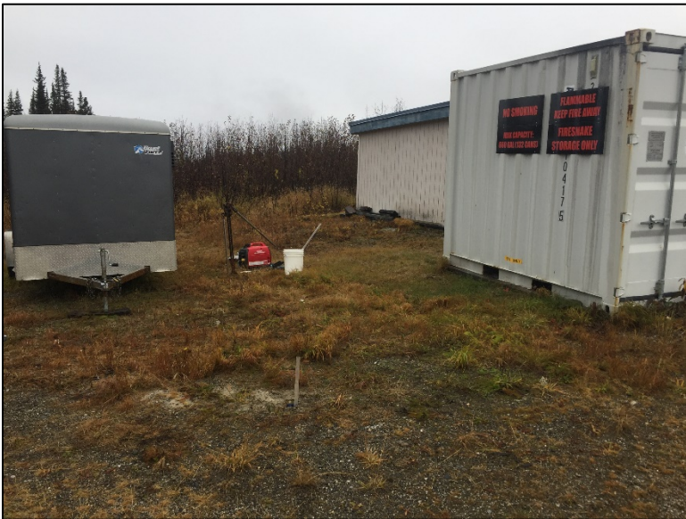
Installing soil boring RSE-8, RSE-7 in foreground, looking south
