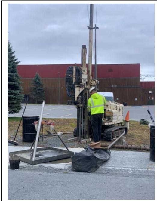
Photo 1: Looking east at the advancement of Boring B1.
