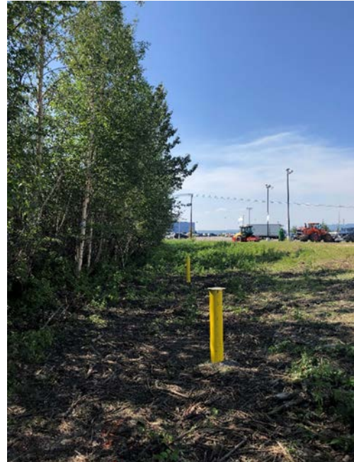
Photo 4: Looking west at completed MW 19-1 (in foreground) and MW 19-2 in protective aboveground steel casings.
