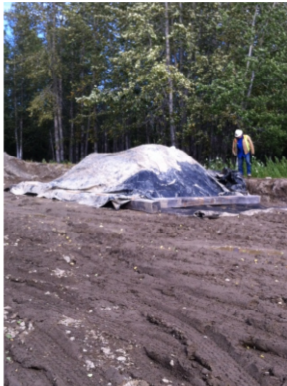
PHOTOGRAPH 4: VIEW OF THE COVERED STOCKPILE, LOOKING NORTH (SEPTEMBER 2012)
