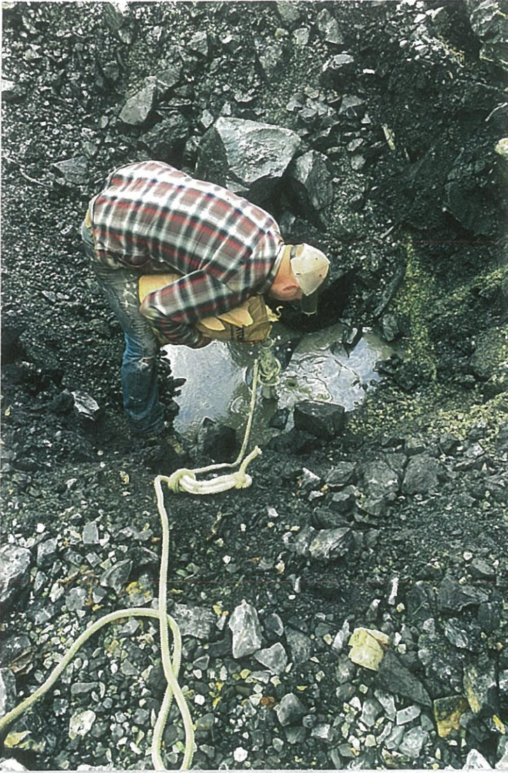
Photo #11: 5/6/20 view of the groundwater well in front of the Phoenix Logging shop, after its initial length and coupler had been removed. Bentonite chips had just been poured into the pipe, then rammed quickly down and out before they could swell and plug the pipe.
