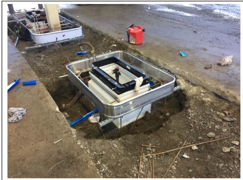
Photo 2: Looking southwest at a diesel fuel dispenser excavation. (November 29, 2018)
