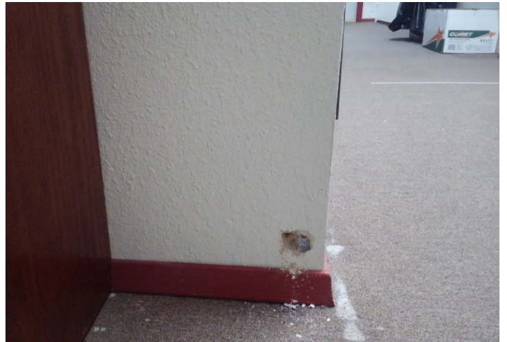
Photo 18. Sample A-6, Hallway Divider Wall, Corner CB, Wall Material
