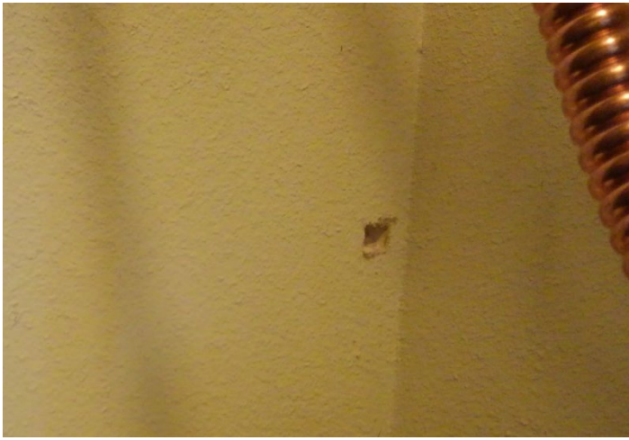
Photo 19. Sample A-7, Storage Room, Corner BC, Wall Material
