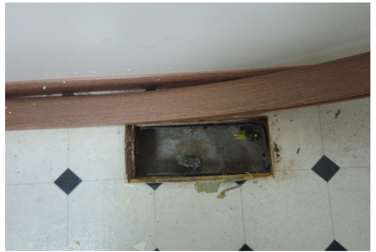
Photo 16. Sample A-4, Bathroom 2, Wall C, Flooring and Mastic
