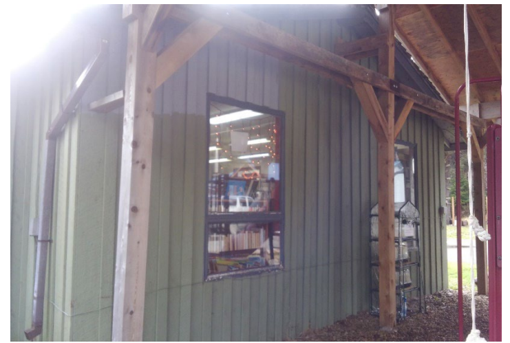
Photo 4. Kasaan Library (facing south-southwest)
