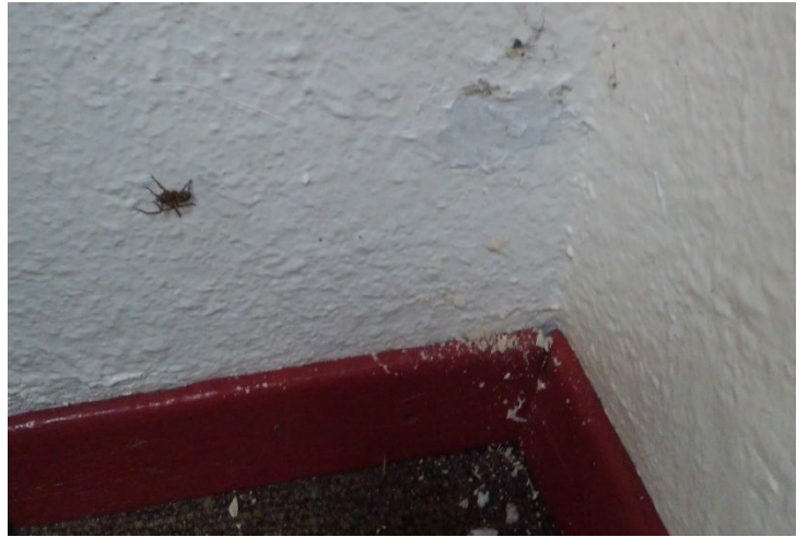
Photo 14. Sample A-2, Library, Corner AB, Wall Material, Post-Patching
