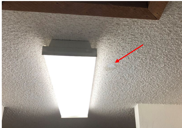
Photo 17. Sample A-5, Hallway, Ceiling, Ceiling Texture
