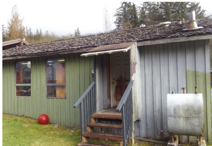
Photo 3. Kasaan Library (facing northeast)
