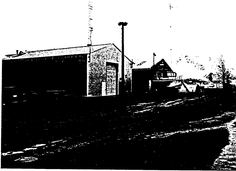
Photograph No. 5: May 8, 1995; Silver and Blue Buildings
