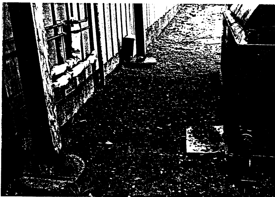
Photograph No. 2: May 8, 1995; Surface soils in vicinity of AST with wrapped pipes next to Blue Building
