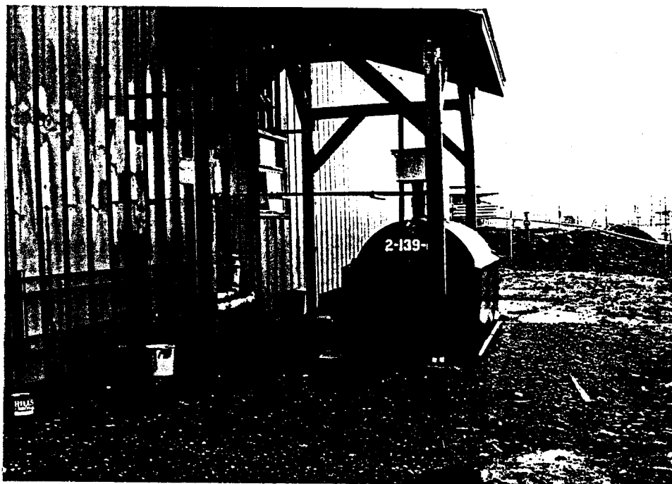
Photograph No. 1: May 8, 1995; Heating oil AST next to Blue Building
