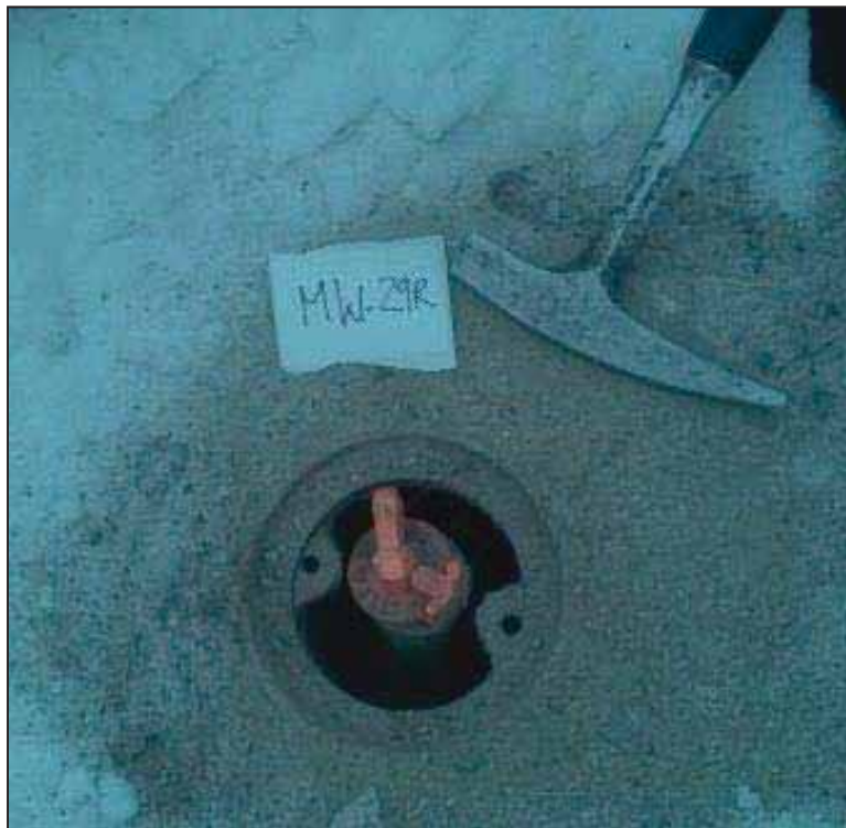
PHOTOGRAPH 14: MW-29R MODERATE CONDITION - CASING IS ALMOST TOUCHING MONUMENT LID - WELL REMOVED APRIL 2014
