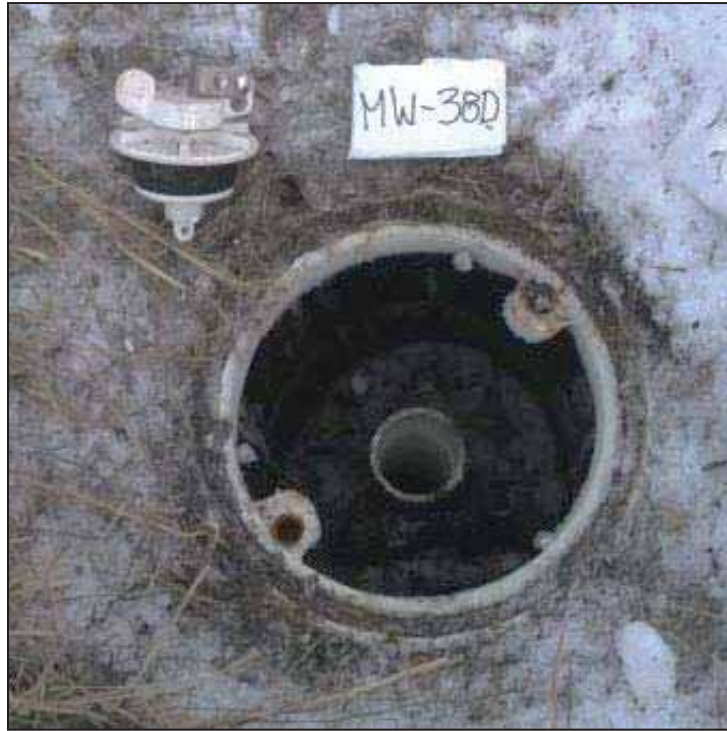
PHOTOGRAPH 23: MW-38D GOOD CONDITION
