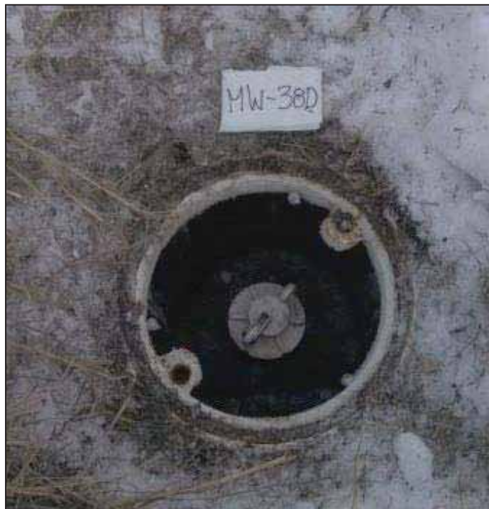
PHOTOGRAPH 22: MW-38D GOOD CONDITION
