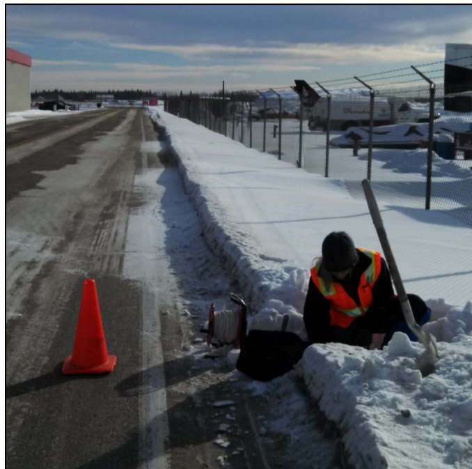
PHOTOGRAPH 4: MW-12 WELL INTEGRITY SURVEY AND DATALOGGER DEPLOYMENT
