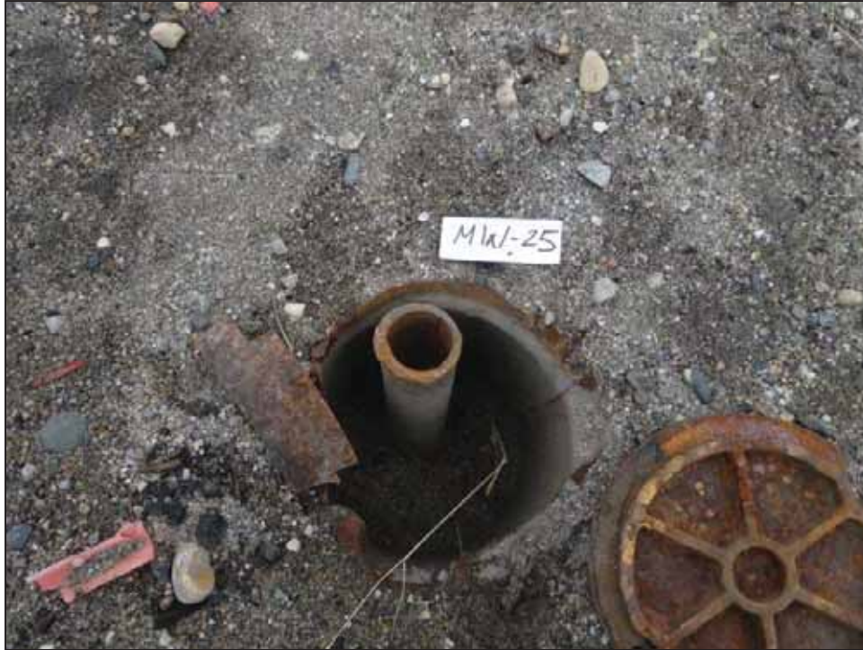
PHOTOGRAPH 13: MW-15 POOR CONDITION - MONUMENT AND CASING HAVE JACKED ABOVE GROUND. MONUMENT LID NOT ABLE TO COVER MONUMENT.
