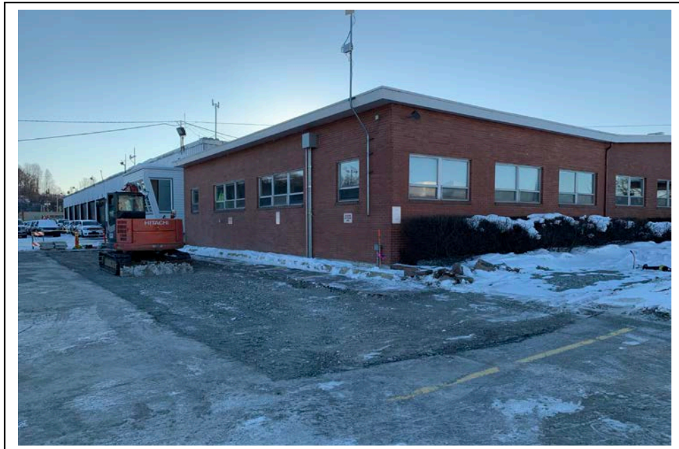
Photo 4: Looking east at the excavation, following backfilling. (March 5, 2020)
