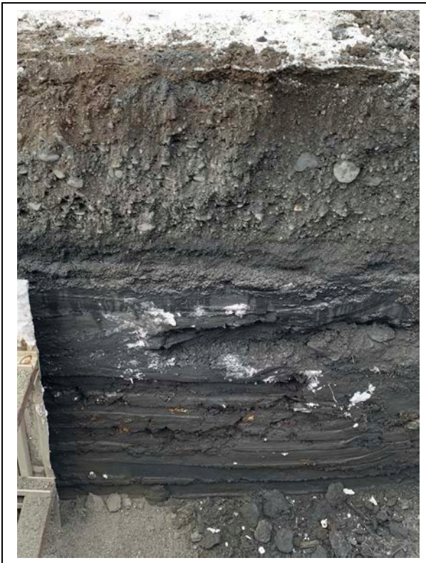
Photo 2: Looking west at the excavation sidewall. Gravel, sand, and silt was present from the ground surface to about 4 to 5 feet bgs. The remainder of the excavation consisted of silt with clay and organics. (February 22, 2020)
