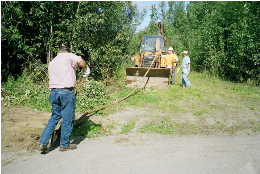
Photo 4. View to north. Removal of the off-site portion of the pipeline extending beneath the adjacent roadway.
