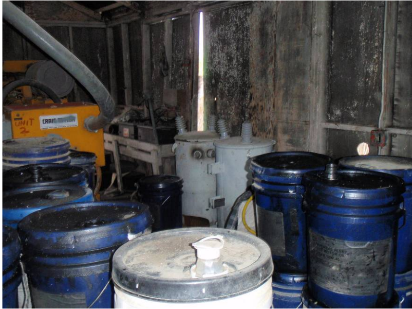
Inside Old Power Plant Building
