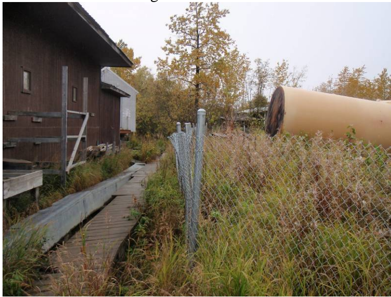
Limited access for test pitting near Old High School Tank Farm
