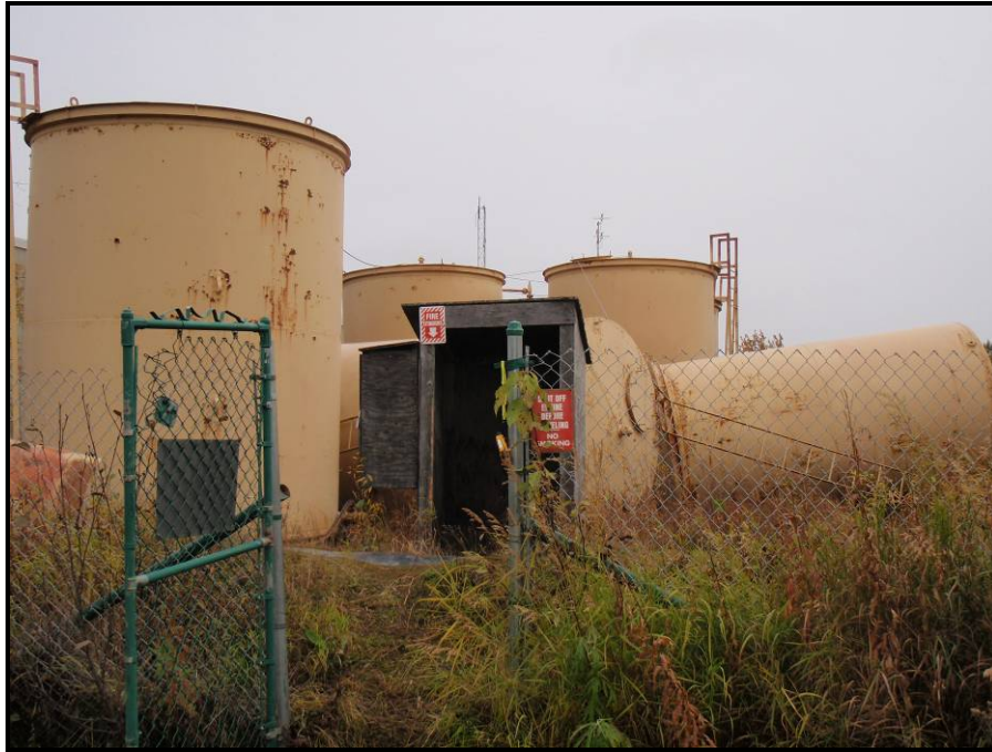
Photograph 1: Old High School Tank Farm as observed during the September 2009 Site Visit. Out of the eight tanks located in the tank farm, three were no longer standing.
