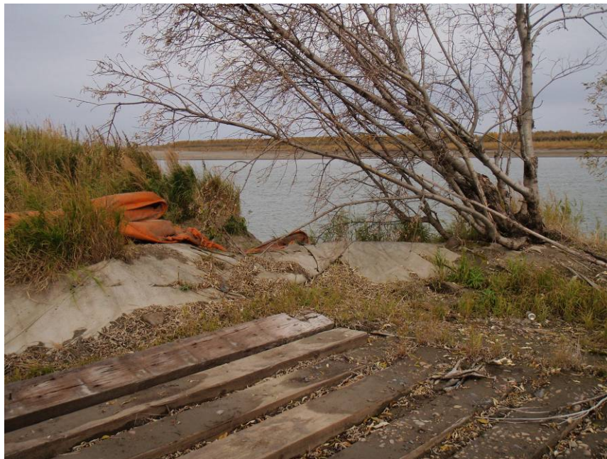
Old Corporation Tank Farm with Kuskokwim River in background
