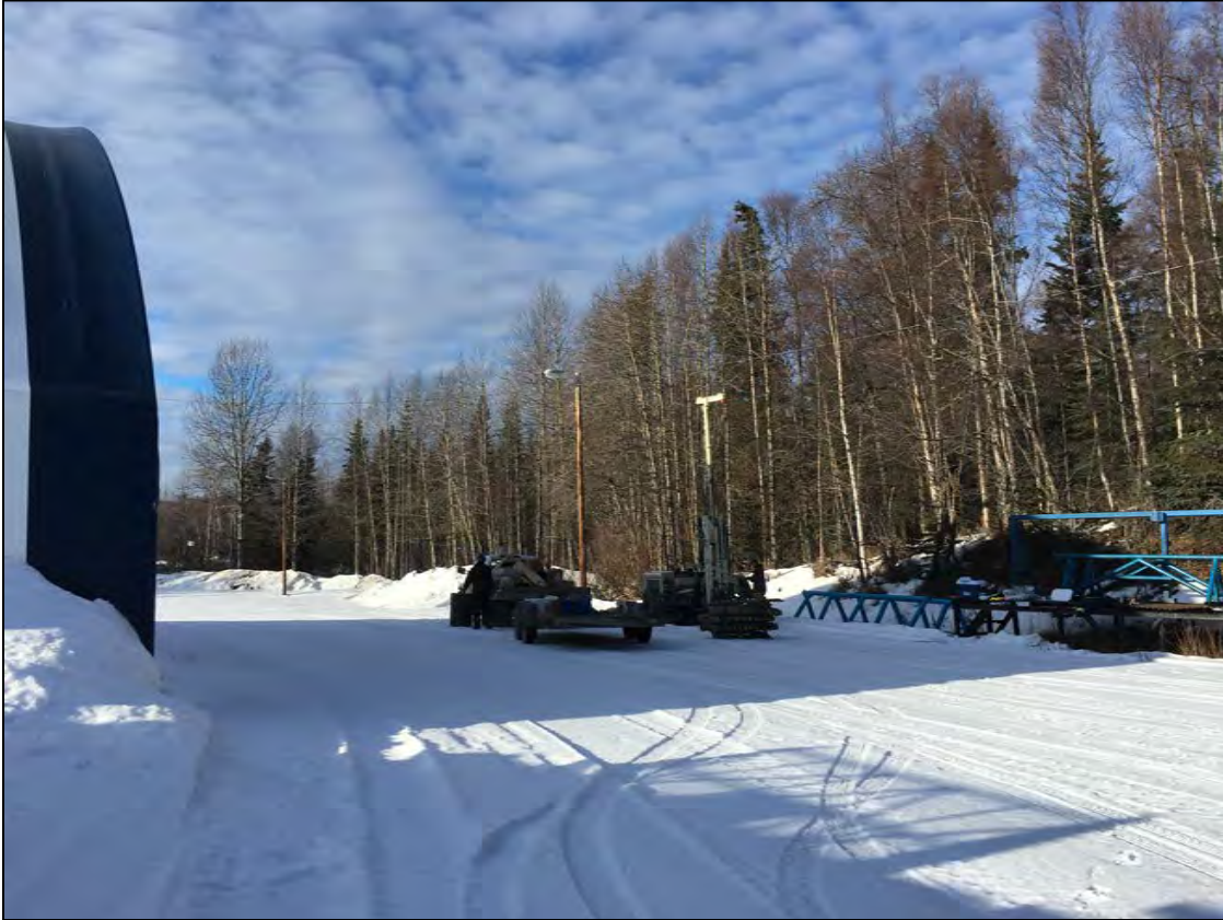
Photo: 5 Time: 1352 Date: 2/15/2016 Direction: West Subject: Drilling at SB-20/MW-20.
