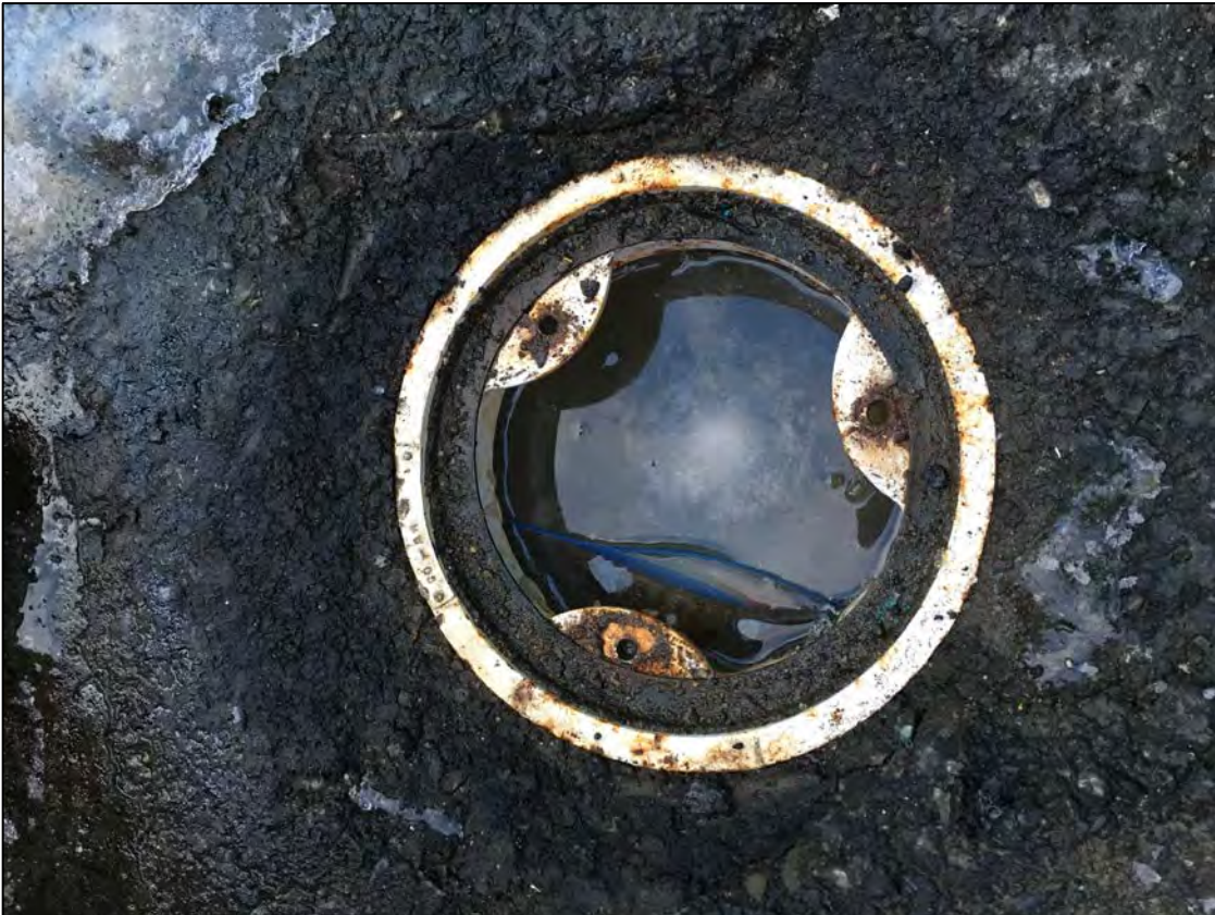
Photo: 8 Time: 1016 Date: 2/15/2016 Direction: Down Subject: MW-05 opened.
