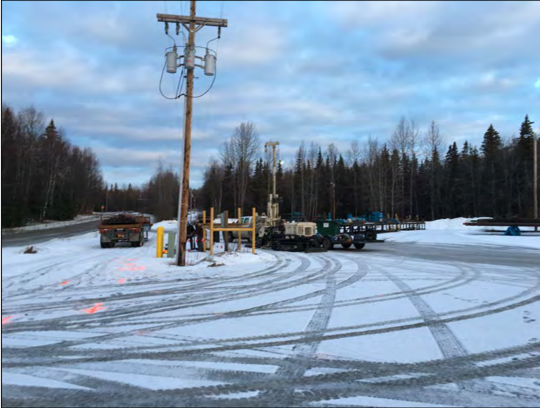
Photo: 3 Time: 1915 Date: 2/15/2016 Direction: West Subject: Drilling at SB-19/MW-09.
