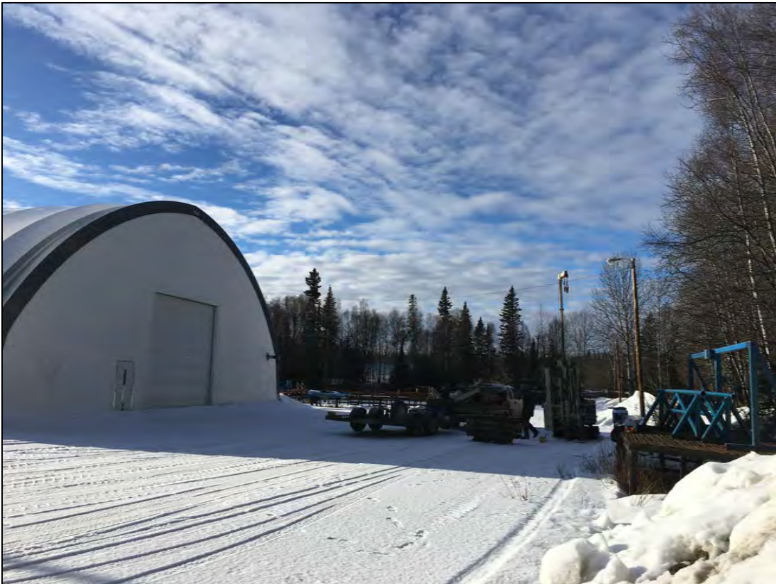
Photo: 6 Time: 1352 Date: 2/15/2016 Direction: West Subject: Drilling at SB-20/MW-20.
