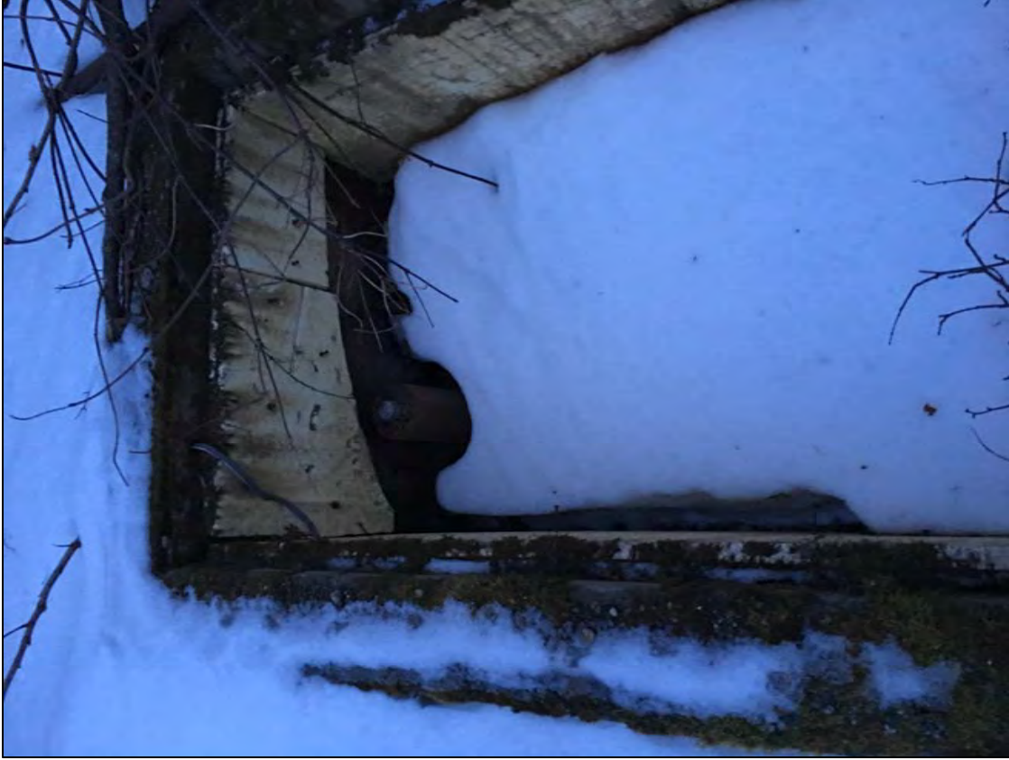
Photo: 11 Time: 1808 Date: 2/14/2016 Direction: East Subject: Old McGahan well head
