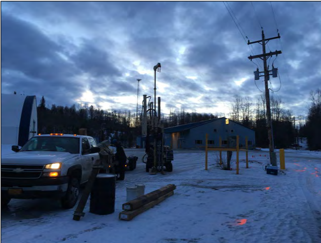
Photo: 4 Time: 0846 Date: 2/15/2016 Direction: East Subject: Drilling at SB-19/MW-09.
