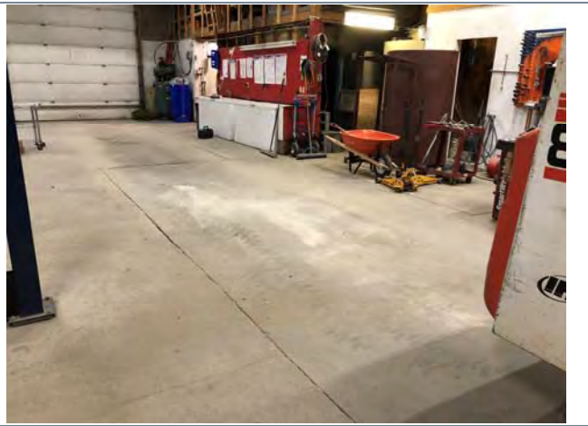
Photo 76: Shop View with Freezers, Facing Southeast
