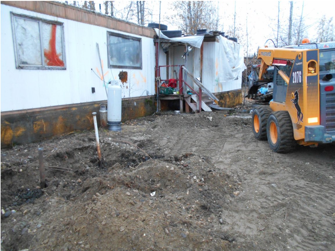
Figure 9. Looking West on October 6, 2013 at soil removal from the path of hydrocarbon transport during snowmelt and rainfall
