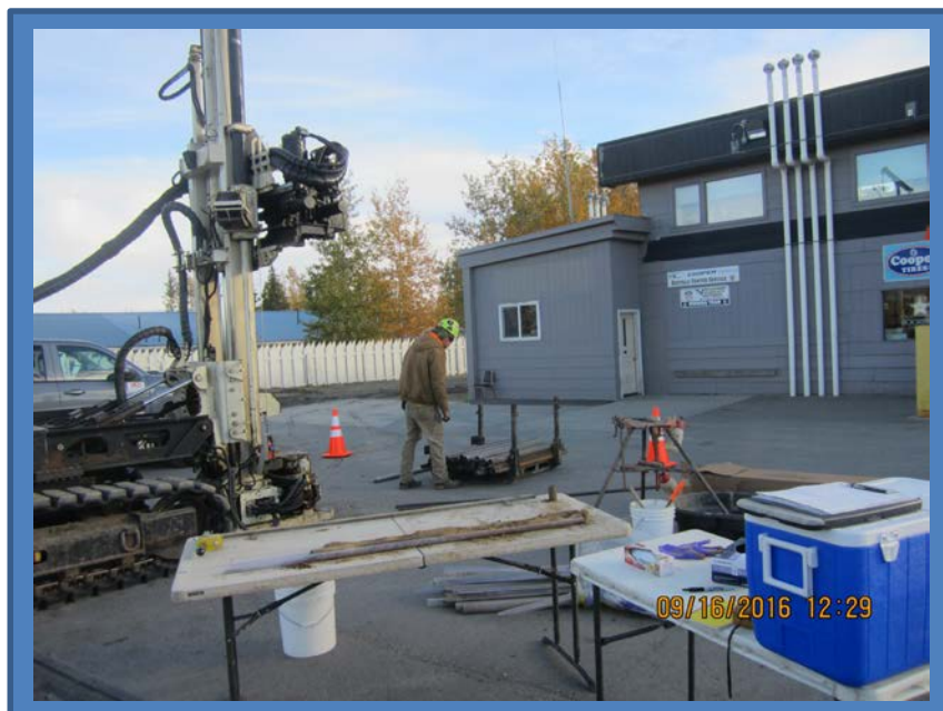
Photo 6: Boring B-6-2016. Temporary well point installed (SP-16). (September 16, 2016)
