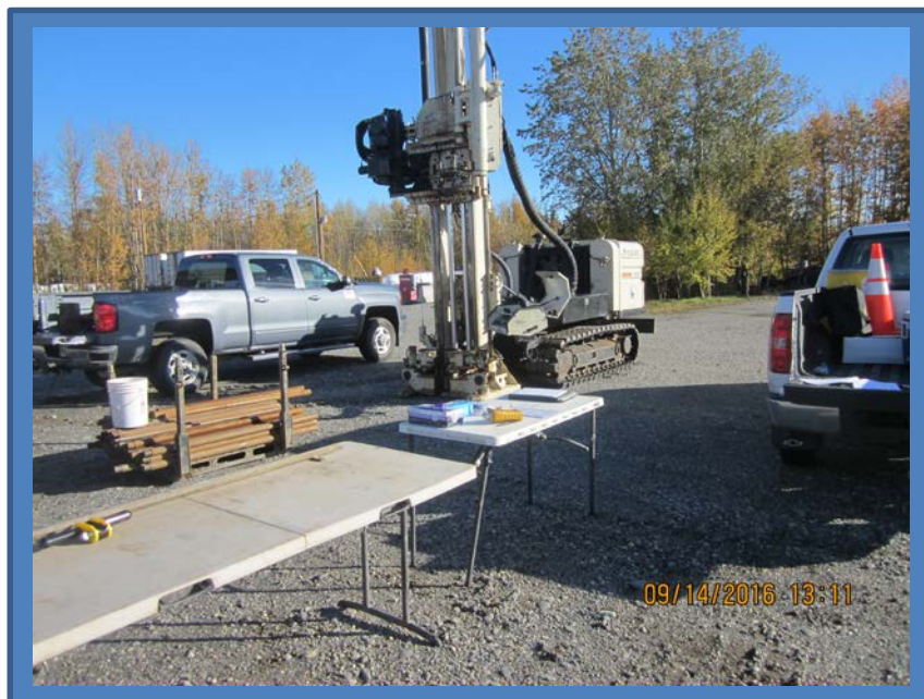
Photo 2: Location of boring B-1-2016. South east side of service station. Temporary Well Installed (SP-16). (September 14, 2016)
