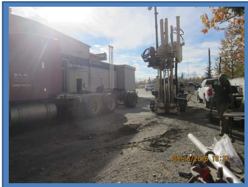
Photo 8: Boring B-8-2016. Located just east of the former tank pit. (September 16, 2016)
