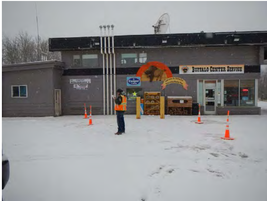
Photo 7: Boring locations IT-B6 , IT-B7 , IT-B9 , and IT-B10 marked by orange cones in front of the Buffalo Service Center. (October 18, 2017)
