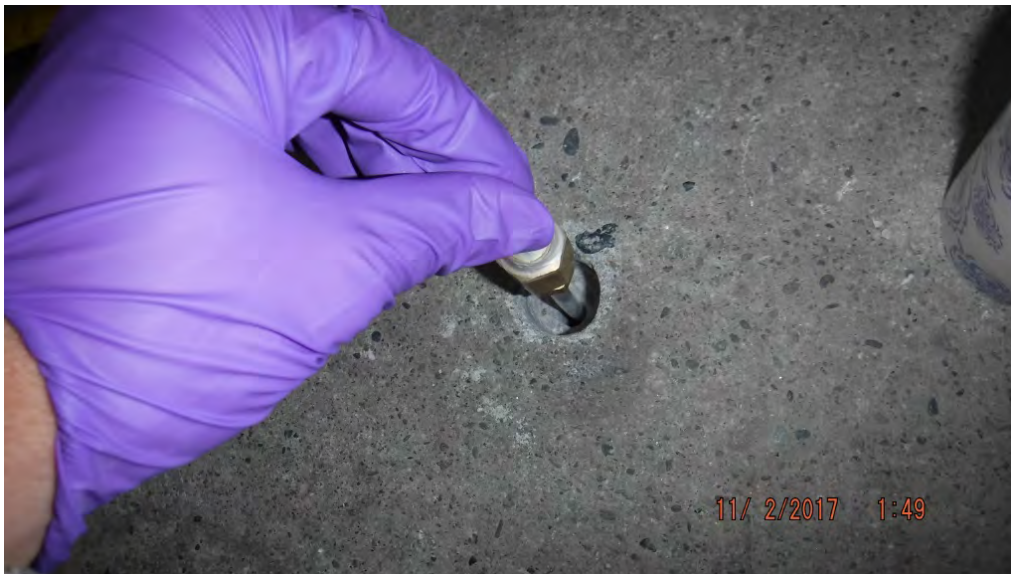
Photo 12: Installing a sub-slab sampling port in the service station garage. (November 2, 2017)
