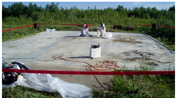
Lead paint is removed from concrete prior to demolition at a site in King Salmon, Alaska
