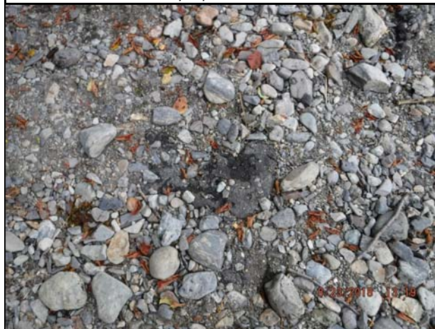
Photo 3 – Asphalt piece lying in gravel. Date: 8/23/18. Time: 1319.
