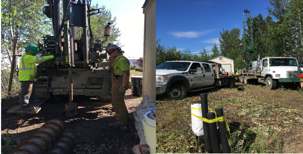
Drilling WRW 2020 Remediation Well on July 14, 2020 at Speedway Store 5313 (former T2GM 101)
