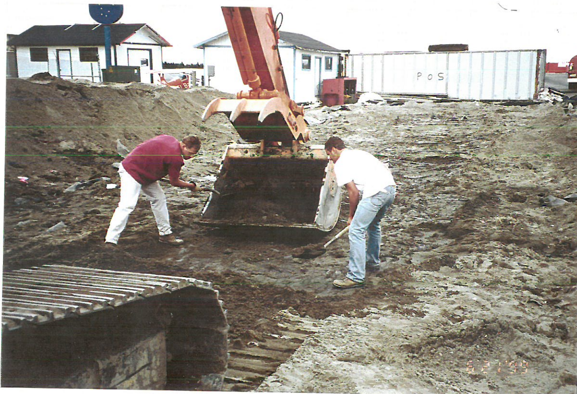
View to west. Cleaning soil off stockpile liner.
