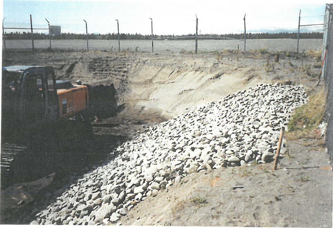
3) View to the Southwest. Drain rock on the North bank to prevent erosion from runoff.
