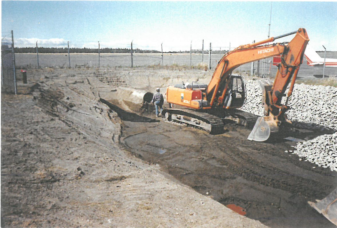
5) View to the Northwest. Pond excavated to groundwater level.
