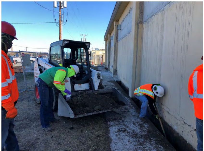
Exhibit 3-1 Field-screening during excavation along the eastern perimeter of B3025.
