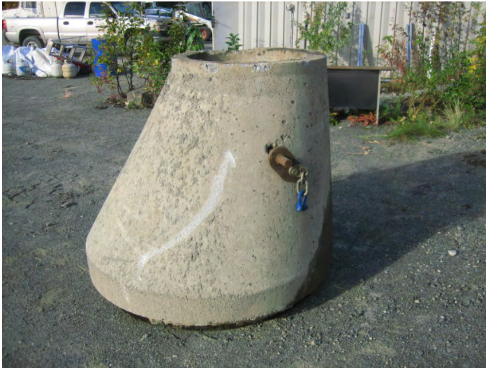
Photo 3: Top section of oil/water separator tank removed
