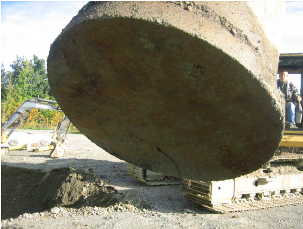
Photo 5: Lifting out base section of oil/water separator tank
