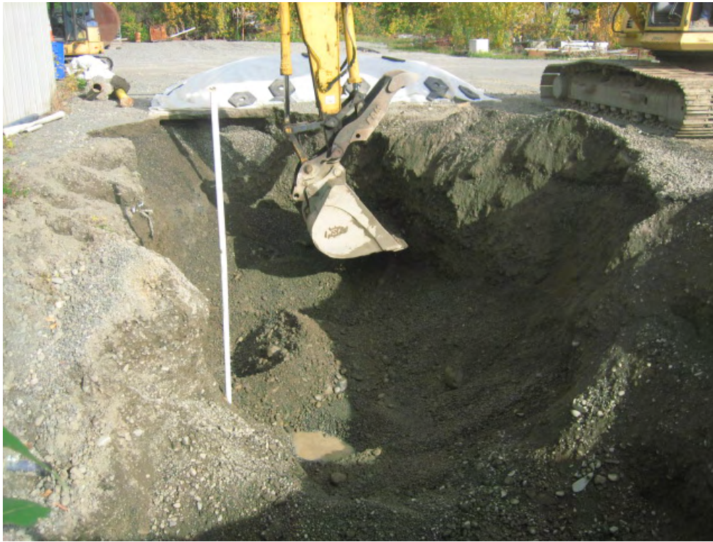
Photo 10: Excavating leachfield, looking north. Monitor Well #1 remains; Monitor Well #2 was removed and decommissioned.
