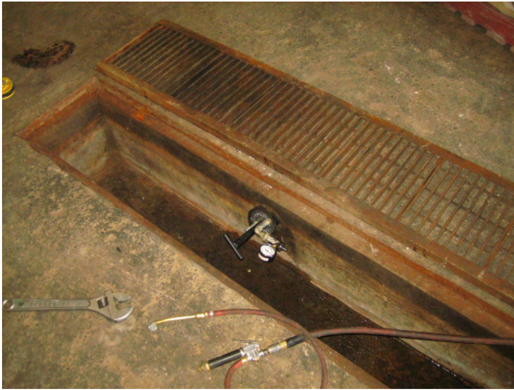
Photo 1: Pressure testing of piping between floor sump and oil/water separator tank
