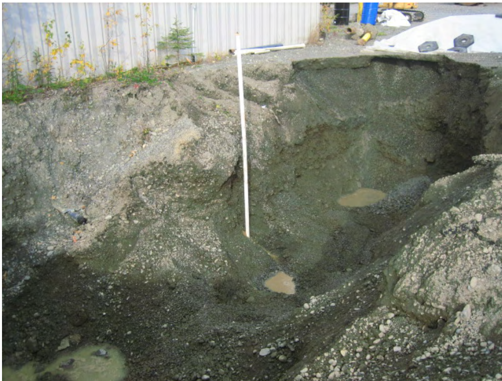
Photo 11: Groundwater observed at approximately 10' below grade. Note undermining of concrete pad near upper right hand corner of photo.
