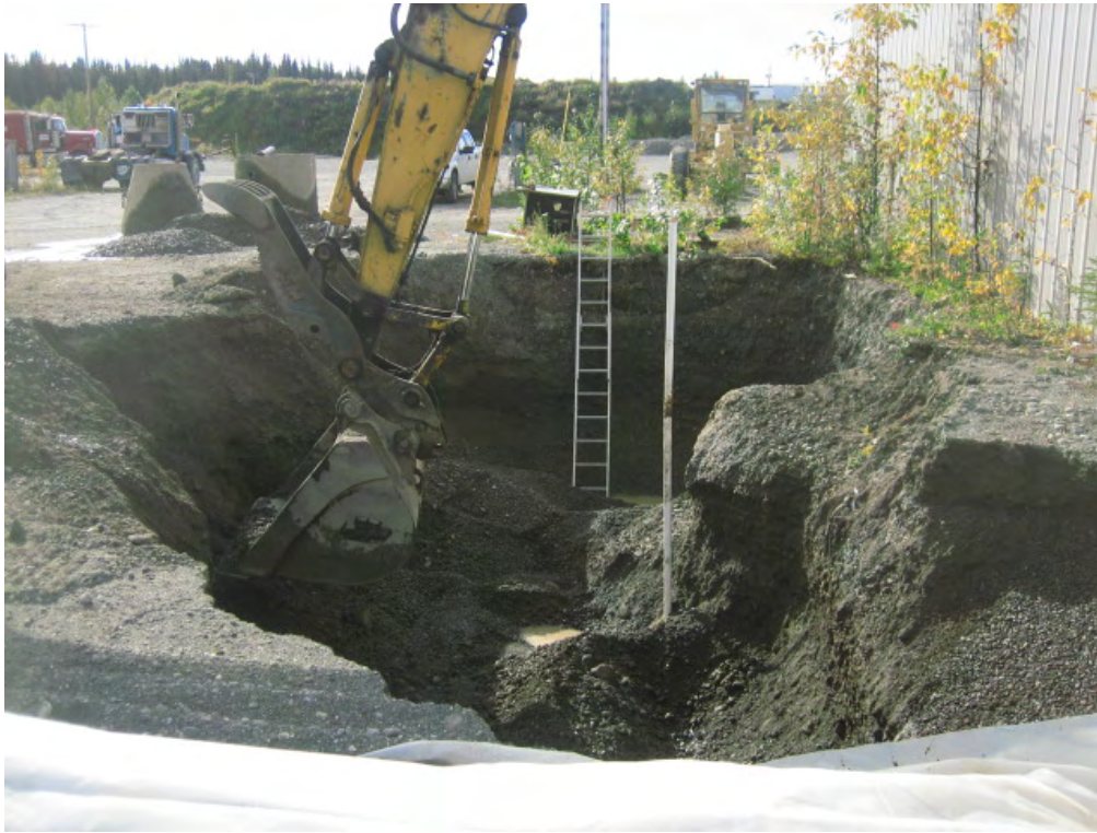
Photo 12: Excavating leachfield, looking south
