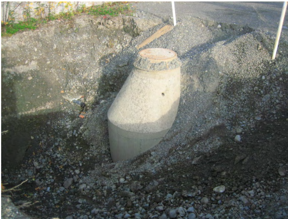
Photo 2: Beginning to excavate oil/water separator tank
