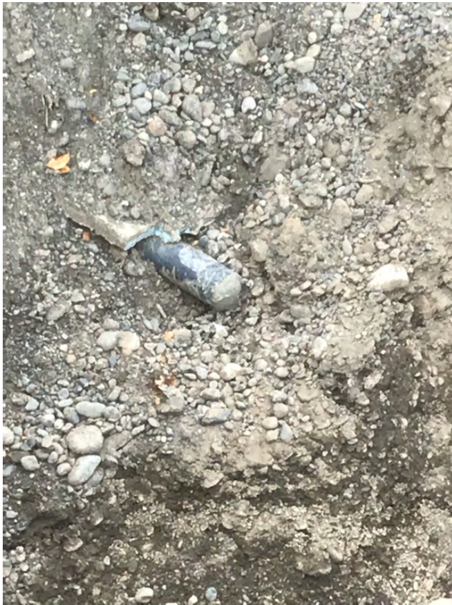
Photo 8: Bentonite slurry was pumped to completely fill piping between floor sump and oil/water separator's previous location (this photo shows exterior end of piping full of bentonite)
