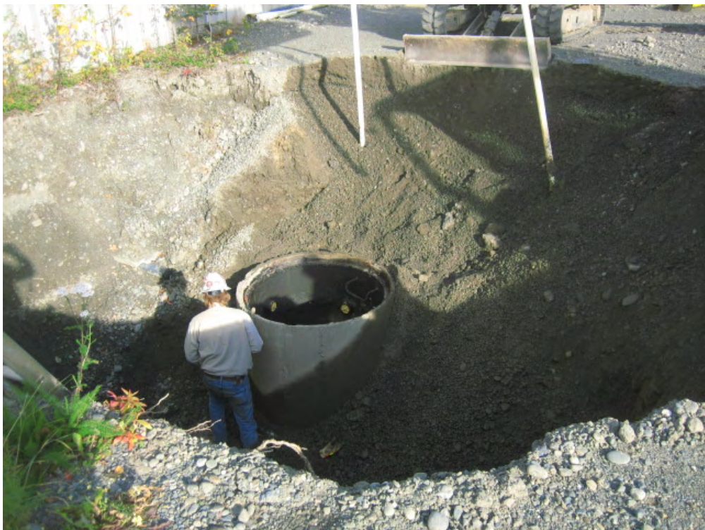
Photo 4: Preparing to excavate base section of oil/water separator tank
