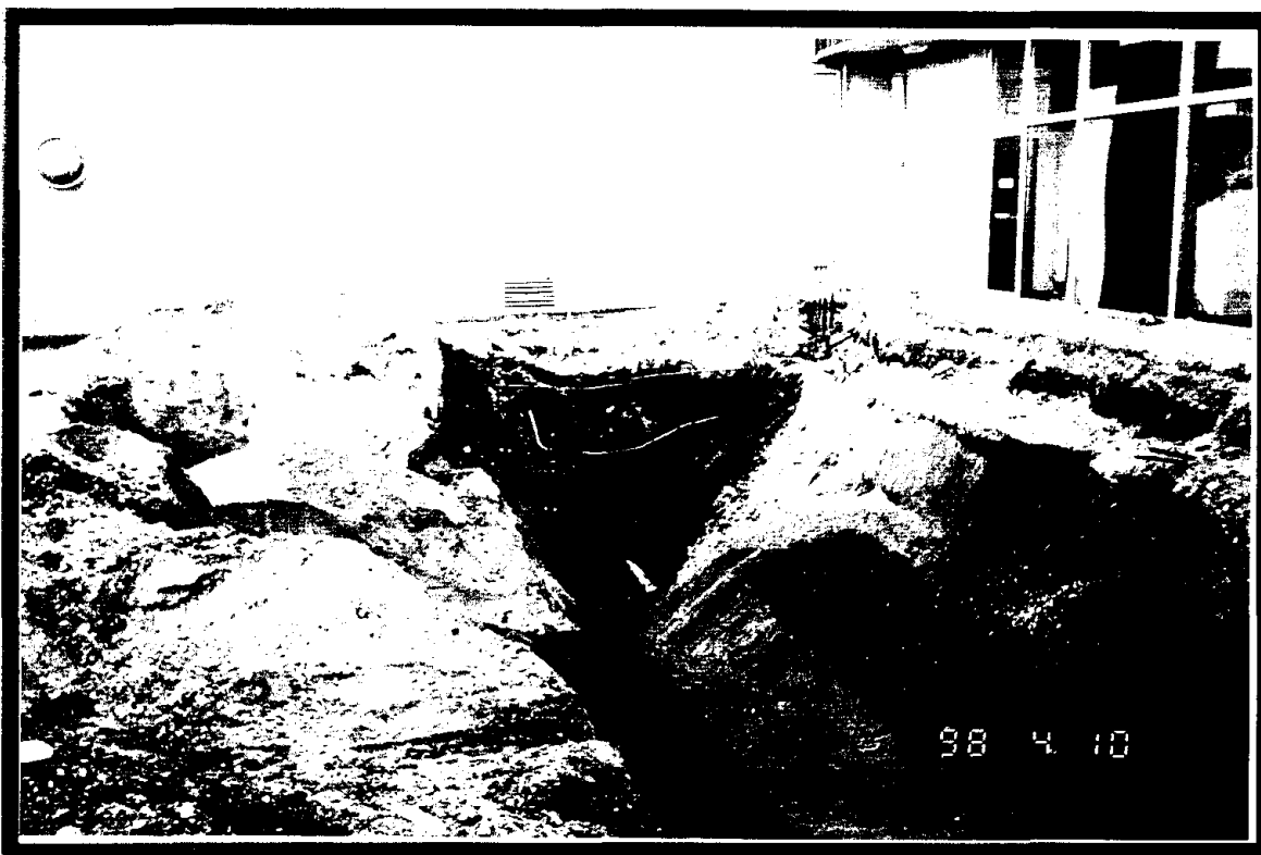
Cline's Tesoro, Anchorage, Alaska Photo 11: Excavation after tanks removed, looking west.
