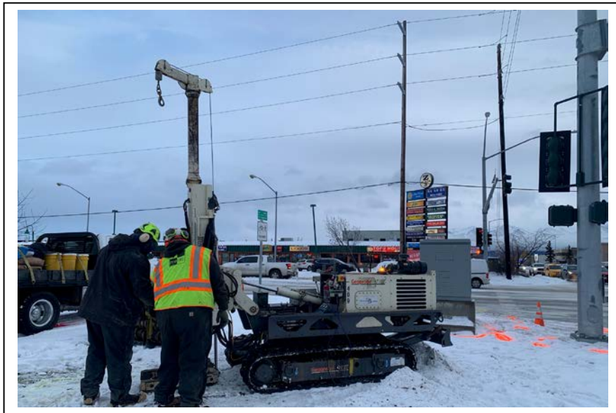
Photo 1: Looking east at the advancement of Boring B5. (December 30, 2019)
