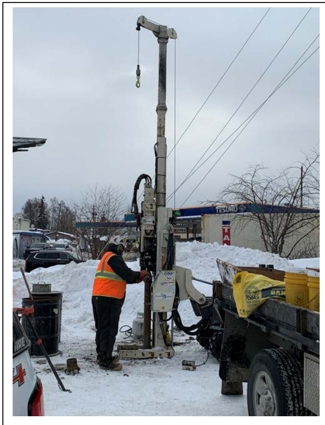
Photo 2: Looking south at the advancement of Boring B7. (February 25, 2020)
