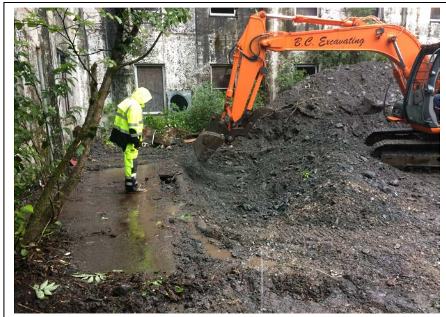
Photo 4: Removing overburden from the tank location. (August 29, 2017)
