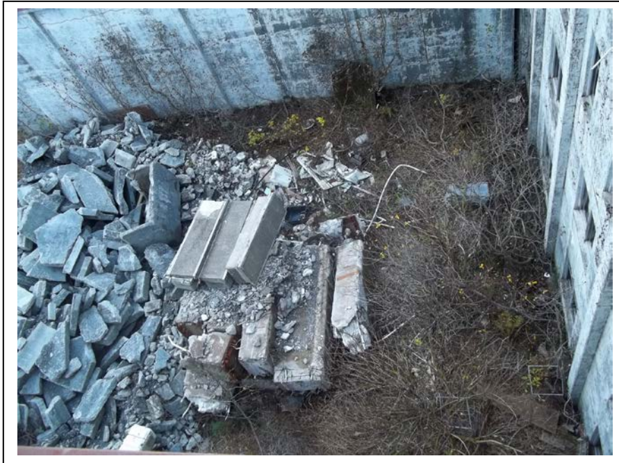
Photo 1: Looking at the location of the UST and concrete and dock debris. (October 22, 2014)
