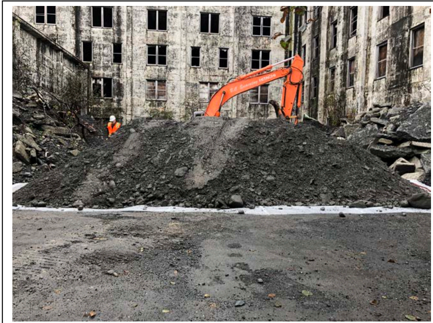
Photo 9: Looking northwest at the stockpiled material. (October 4, 2017)
