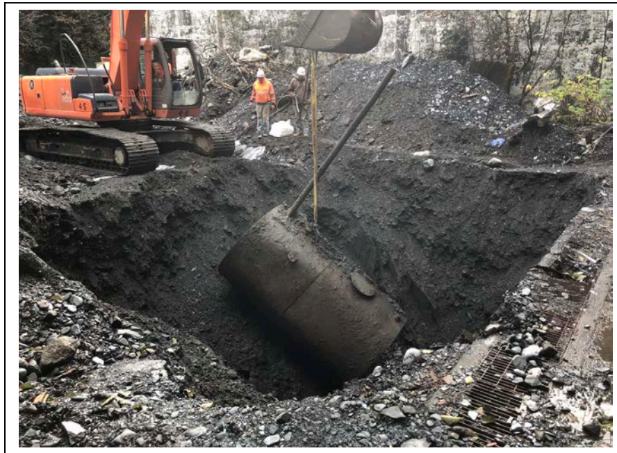
Photo 8: Looking south while removing the UST from the excavation. (October 4, 2017)
