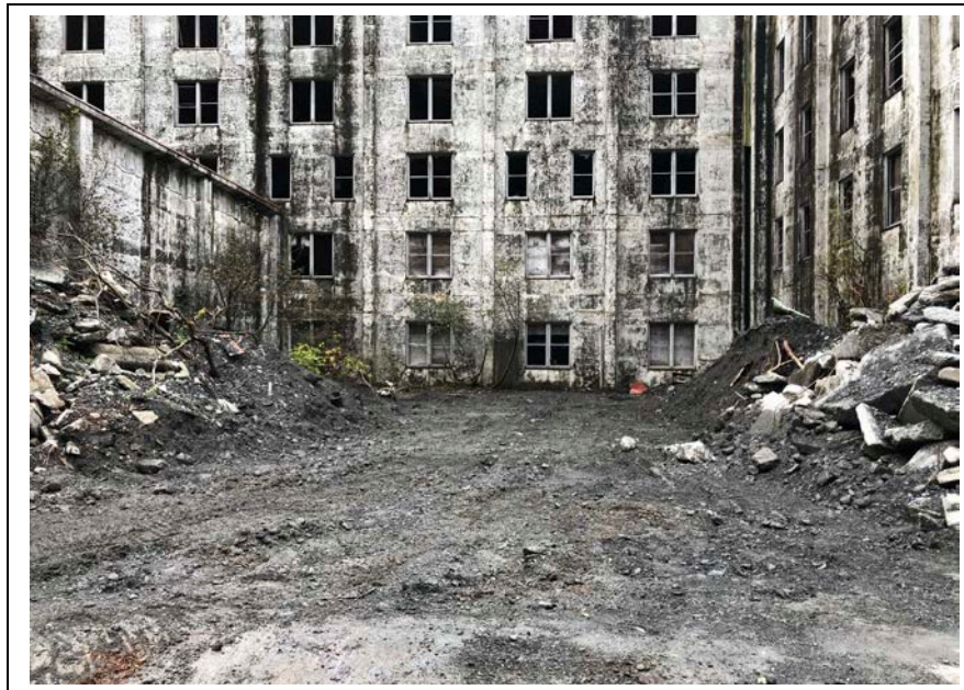
Photo 10: Looking northwest following backfilling. (October 4, 2017)
