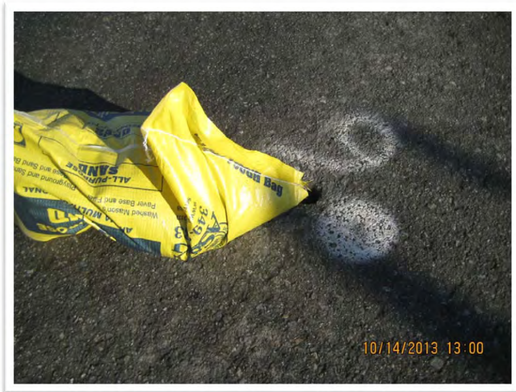
Photograph 9 – After sampling was completed, each hole was backfilled with sand.
