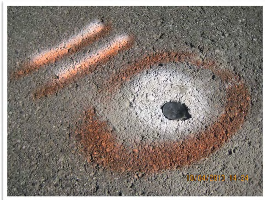
Photograph 7 – Black stoppers were installed below grade in the active parking lot.
