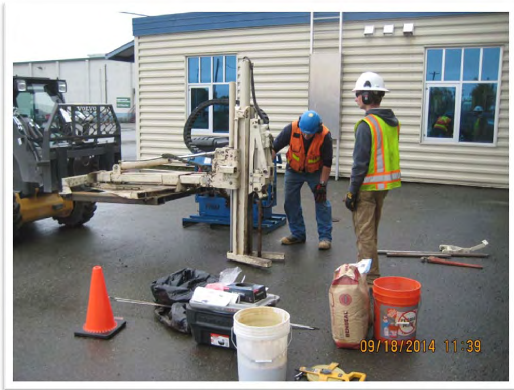
Photograph 3 – Boreholes were installed using percussive techniques. View to the northeast.
