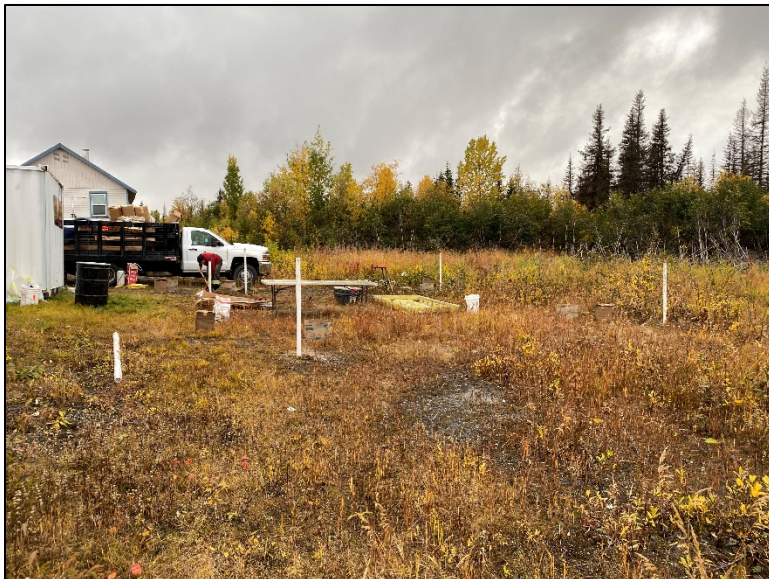
Installing monitoring wells RSE-11, RSE-12, RSE-13, RSE-14 and RSE-15; looking south
