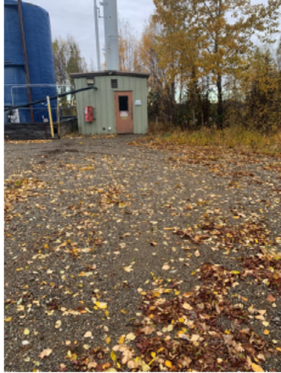
Well 224-13-2 to the right of green facility Facing West
