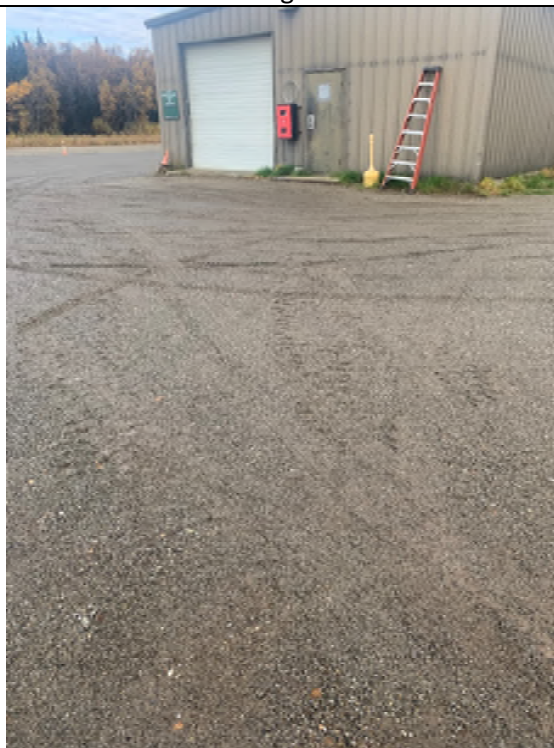
Assumed former location of HOS-6 Facing North
