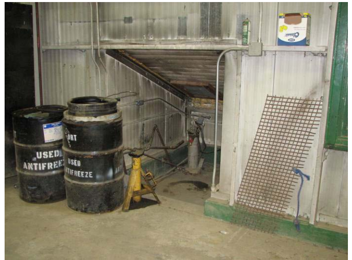
NMS well head; not severed pipe near center of photograph.
