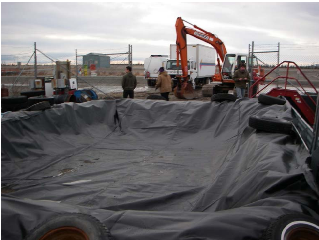
Photo: 13 Time: 1329 Date: 12/29/200 Direction: West Subject: Stockpile containment; loading in 20-mil liner.
