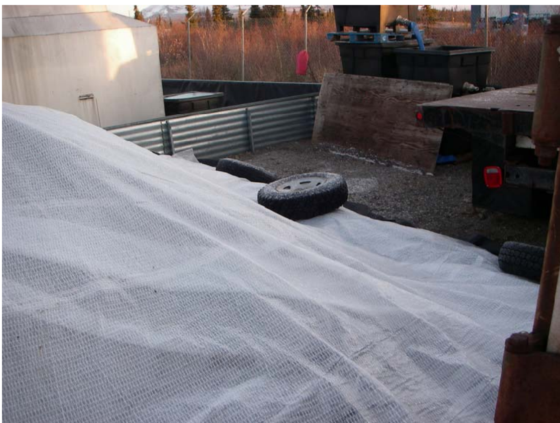
Photo: 70 Time: 1059 Date: 12/31/200 Direction: Northeast Subject: Soil stockpile with 6-mil reinforced cover.
