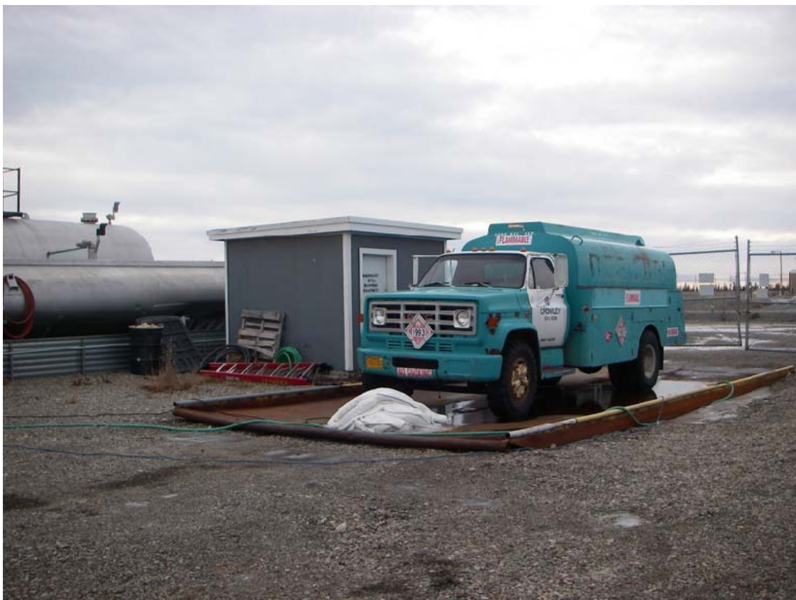
Photo: 17 Time: 1331 Date: 12/29/200 Direction: Southwest Subject: Fuel truck loading deck containment area.
