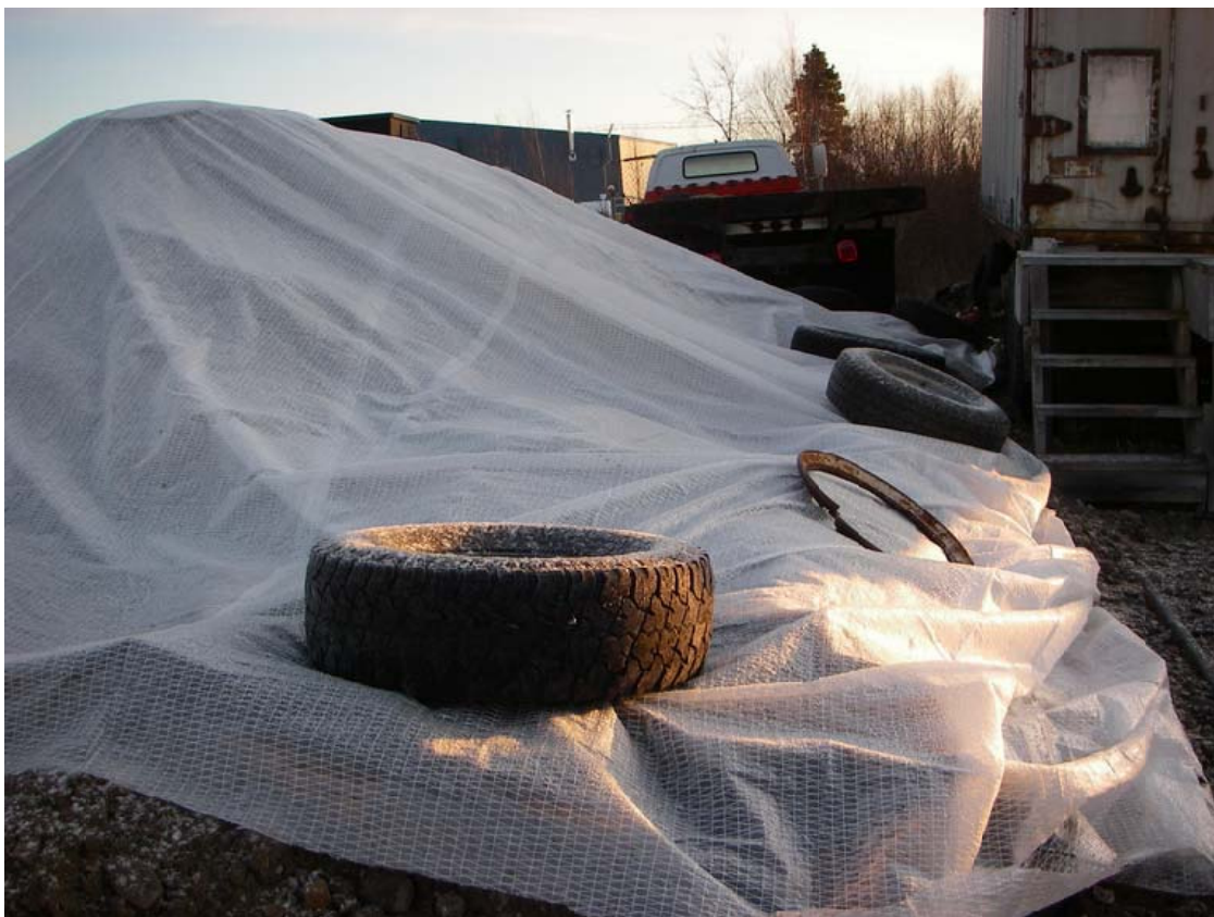
Photo: 69 Time: 1059 Date: 12/31/200 Direction: East Subject: Soil stockpile with 6-mil reinforced cover.
