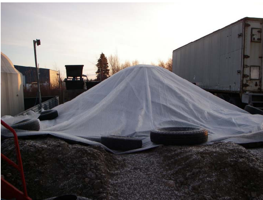
Photo: 68 Time: 1058 Date: 12/31/200 Direction: East Subject: Soil stockpile with 6-mil reinforced cover.
