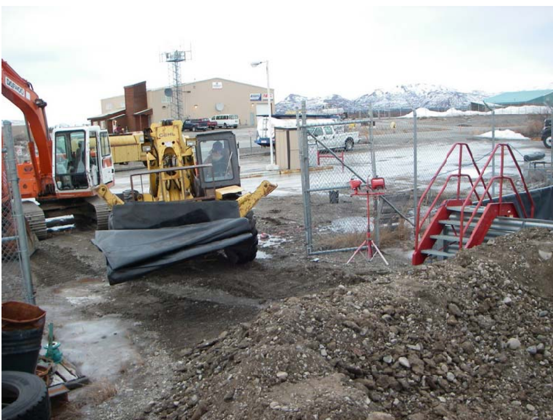
Photo: 12 Time: 1318 Date: 12/29/200 Direction: West Subject: Stockpile containment; loading in 20-mil liner.
