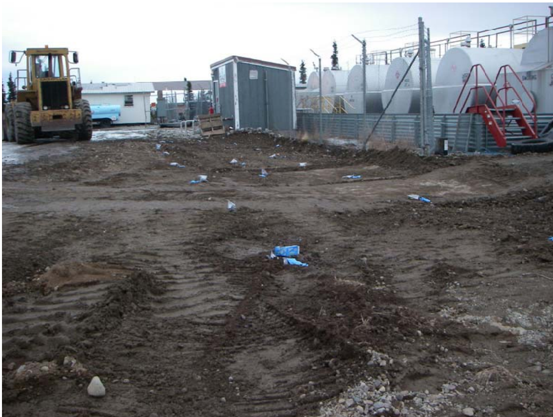
Photo: 45 Time: 1405 Date: 12/30/200 Direction: North Subject: Final excavation extent/depth. PID sample locations 1 through 16 visible.
