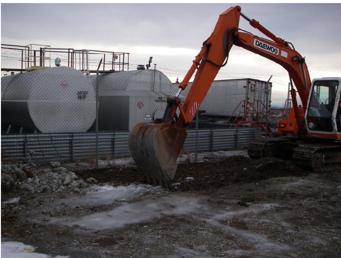
Photo: 18 Time: 1335 Date: 12/29/200 Direction: East Subject: Begin initial removal at fuel spill location.
