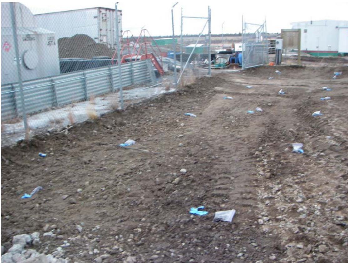
Photo: 43 Time: 1404 Date: 12/30/200 Direction: South Subject: Final excavation extent/depth. PID sample locations 1 through 16 visible.
