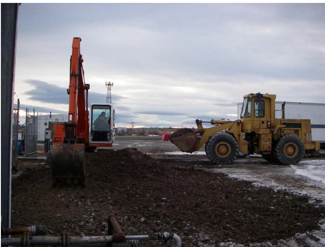
Photo: 20 Time: 1419 Date: 12/29/200 Direction: South Subject: Excavation area. Soil loaded into loader for transfer into the stockpile containment.
