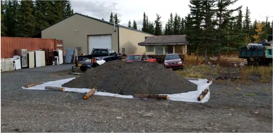
Photo 7: September 17, 2019, looking south - This photo shows the presumed contaminated stockpile. The pile was covered with six-mil polyethylene sheeting after characterization sampling.
