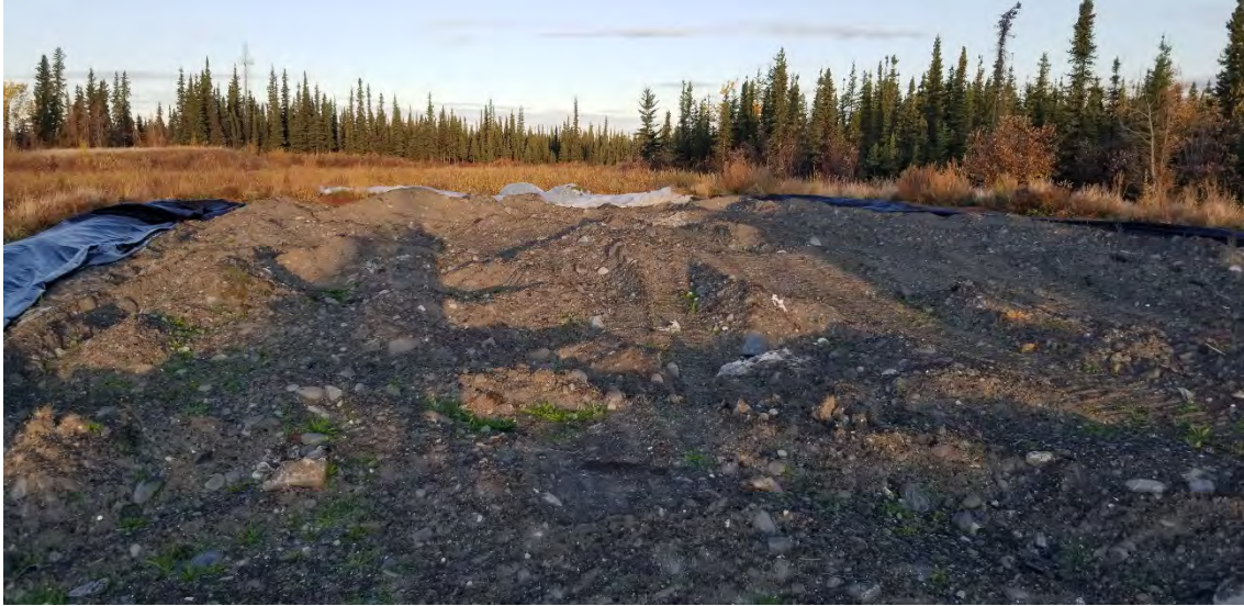
Photo 1 (9/19/2019 - looking west): This photo shows the landfarm prior to characterization sampling. Soil depths throughout the stockpile varied from 1.5 to three feet.
