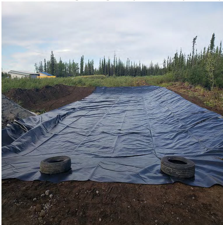
Photo 4: Area of landfarm with liners, facing west. (July 2018)
