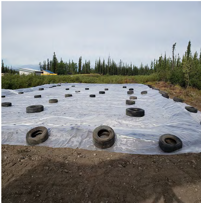
Photo 6: Covered landfarm, facing west. (July 2018)
