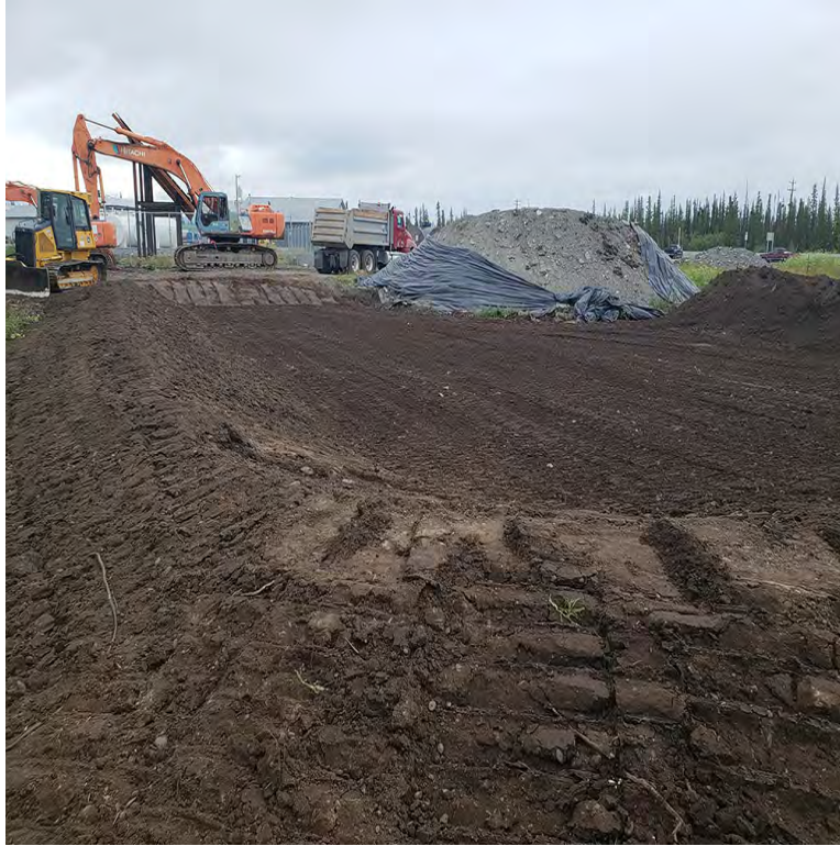
Photo 3: Area of landfarm prior to spreading of soil, facing east. (July 2018)
