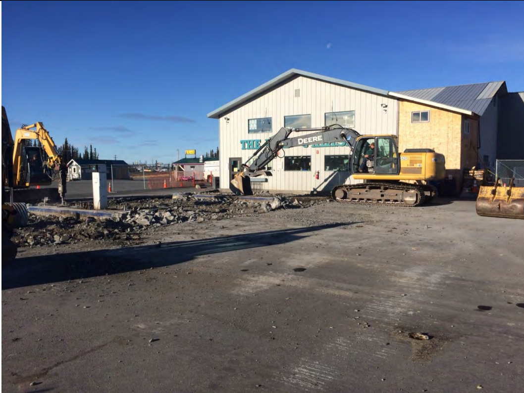
Photo 1: Dispenser area during slab removal; looking southwest. First Fuel Island next to the building and the middle fuel island. Satellite diesel dispenser to the left is not shown. (10/9/2017)
