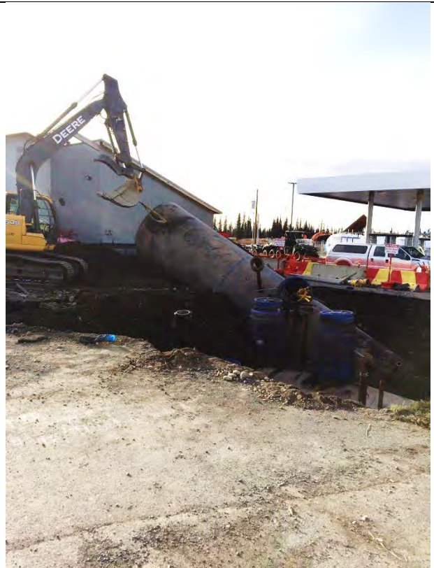
Photo 8 UST #3 being pulled out of the excavation pit. (10/10/17)
