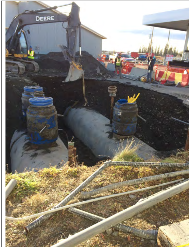
Photo 7 UST #3 prepared for lifting out of the excavation. Looking southwest (10/10/17)
