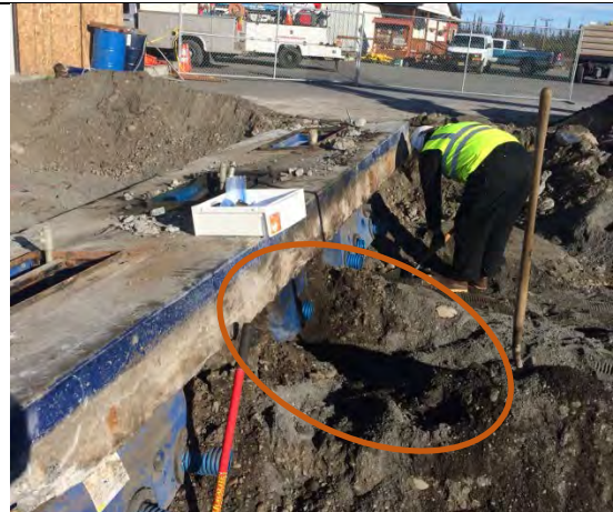
Photo 4 Collecting samples under the dispenser sumps. Contamination was found under the middle dispenser. (10/9/17)
