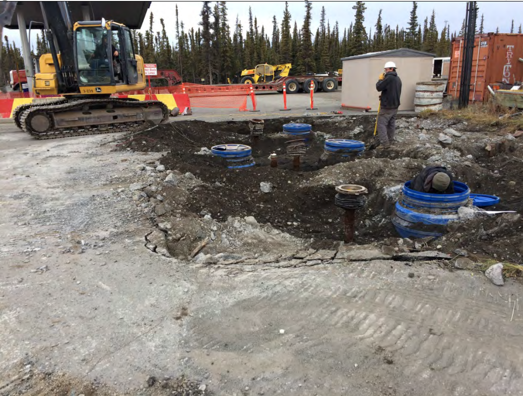
Photo 2: UST area after concrete slab removal; looking west. Shows sumps and fill ports of tanks #1, #2 and #3 going from top to bottom of the picture. (10/10/2017)
