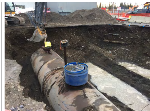
Photo 11 UST #3 being prepared to pull out of the excavation pit (10/10/17)
