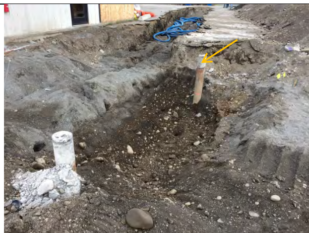
Photo 13 Initial excavation for release at first fuel island. Piles (arrow) were used to measure sample locations. (10/10/17)
