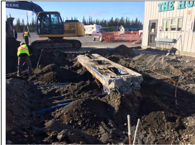
Photo 3 Start of excavation of first dispenser island. Fuel odor noticed at middle dispenser. (10/9/17)
