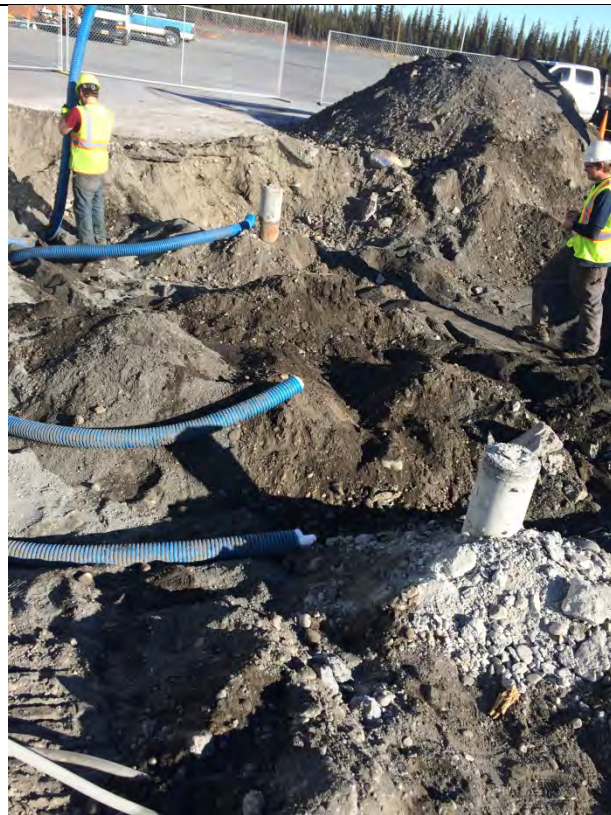
Photo 5 After removal of dispenser island 1 and fuel lines leading to the second dispenser. Looking South (10/9/17)
