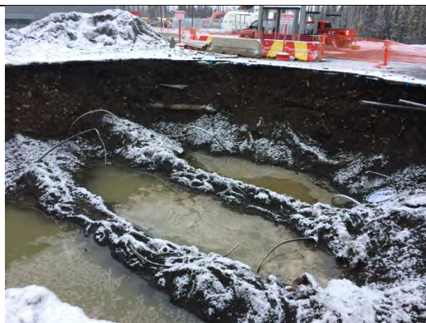
Photo 12 Note the higher water in the excavation bottom the next morning (10/11/17)
