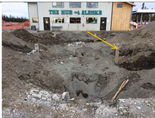
Photo 14 Shows excavation for all three fuel islands. Piles were used to measure sample locations. (10/10/17)
