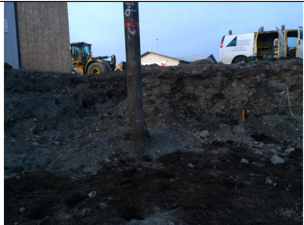
Photo 6 Sidewalls of the excavation. Looking Northwest (10/22/17)
