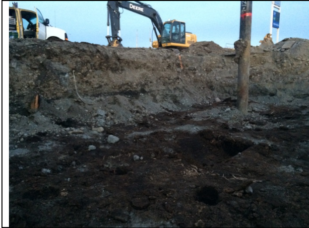
Photo 7 Sidewalls of the excavation. Looking Northeast (10/22/17)
