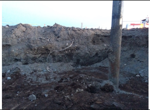
Photo 8 Sidewalls of the excavation. Looking Southeast (10/22/17)
