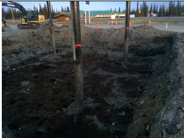
Photo 5 Peat layer on the bottom of the excavation. Looking Northeast. (10/22/17)
