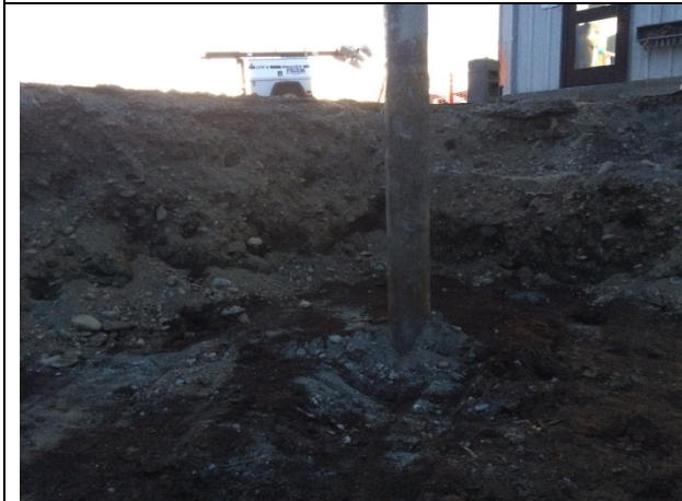
Photo 9 Sidewalls of the excavation. Looking Southwest (10/22/17)
