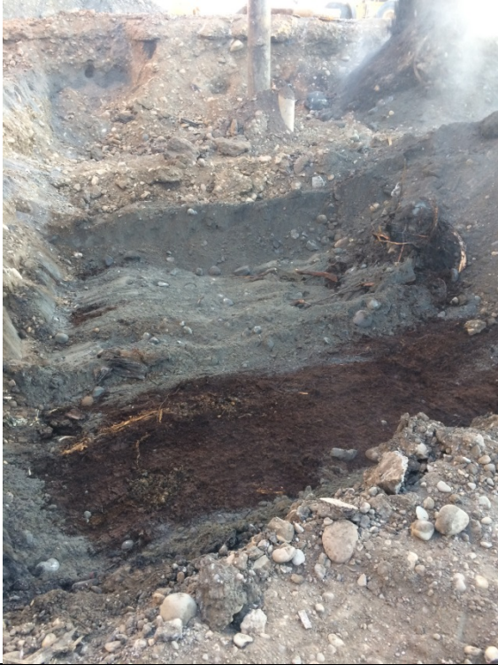
Photo 3 Peat layer found under the layer of sandy fill. Looking North (10/21/17)
