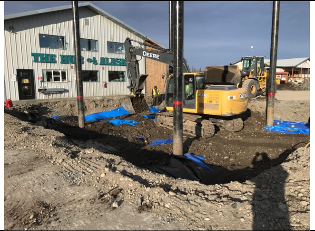
Photo 14 Looking Northwest. Dirt from the segregated and sampled stockpile being placed on the plastic tarp. (10/24/17)
