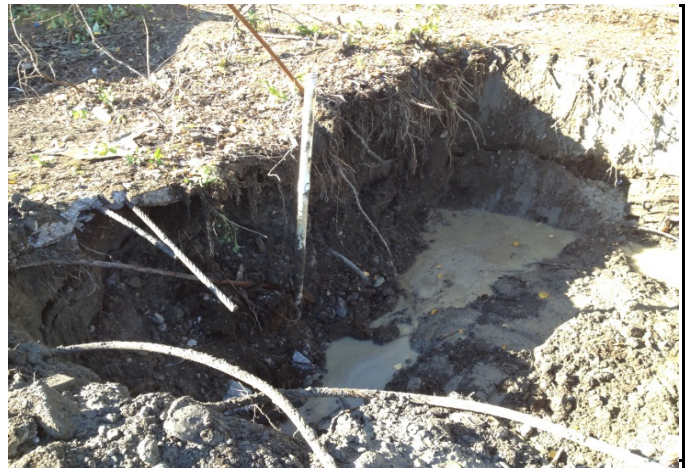
Photo 12. Continued excavation. MW-1 in foreground. 9/22/2014
