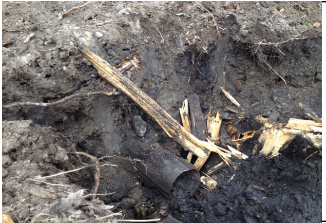
Photo 7. Drill shop sump initial excavation showing drain line to covered pit. 7/15/2014
