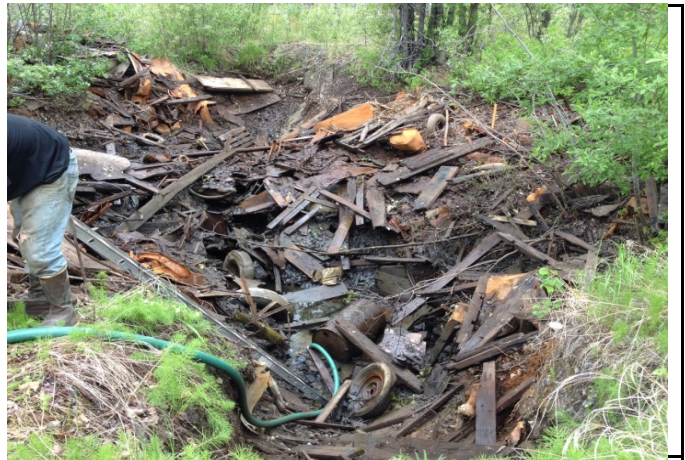
Photo 2. Dewatering open pit. 6/7/2014
