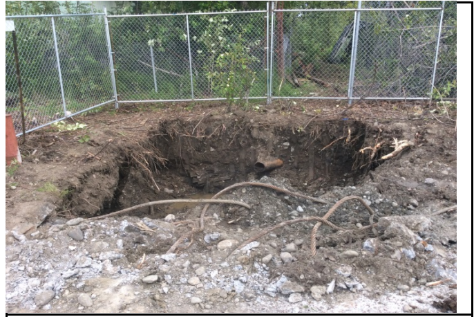
Photo 8. Drill shop sump excavation. Note timber cribbing. 7/16/2014
