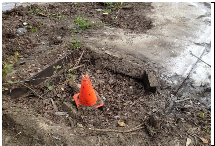
Photo 6. Drill shop sump prior to excavation. 7/15/2014
