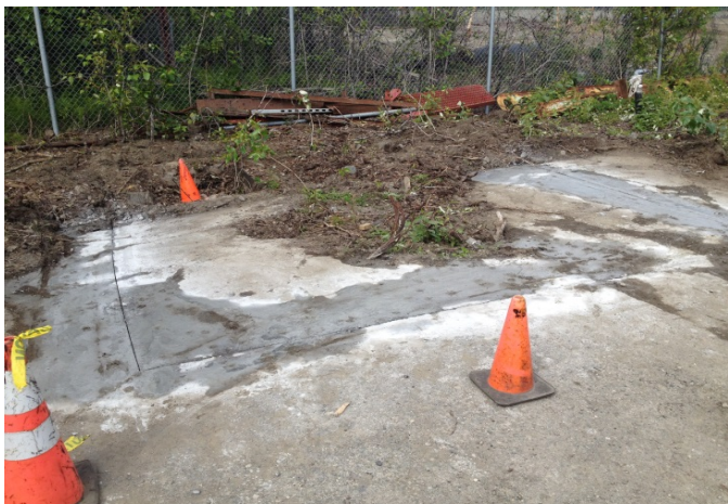
Photo 5. Drill shop sump area prior to excavation. 7/15/2014
