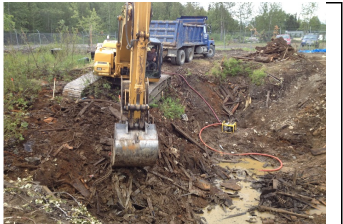
Photo 4. Open pit, debris removal. 7/7/2014
