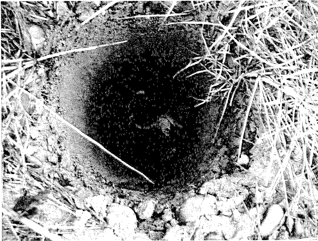
Photograph 2: Broken casing in ground, GW-1.
