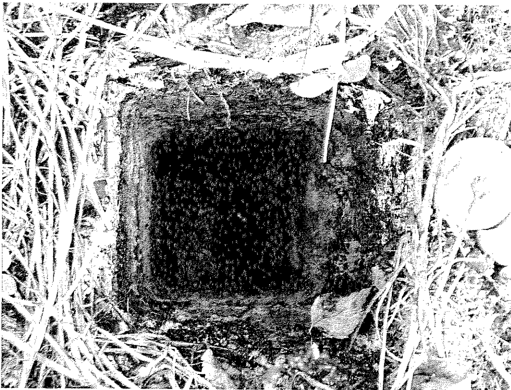
Photograph 5: Remaining hole in B-11MW after with casing removal..
