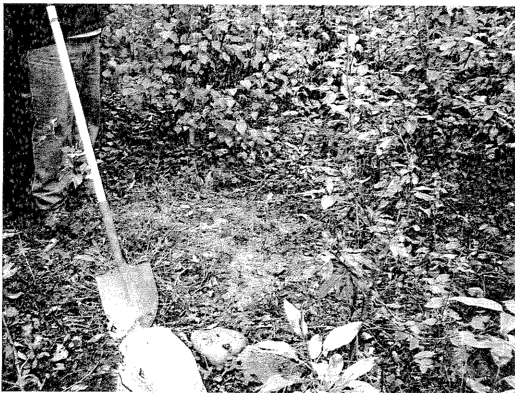
Photograph 6: B-11MW decommissioning completed.
