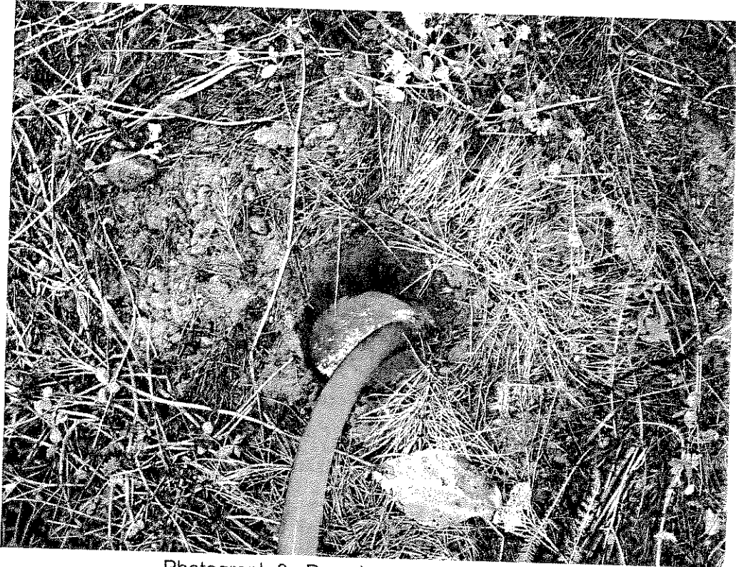
Photograph 3: Pumping volclay into GW-1.
