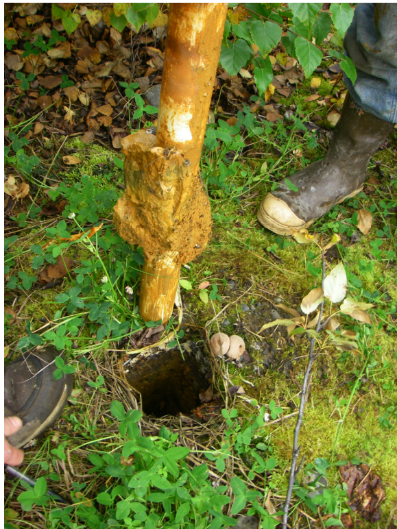
Photograph 4: Removing well casing from B-11 MW.
