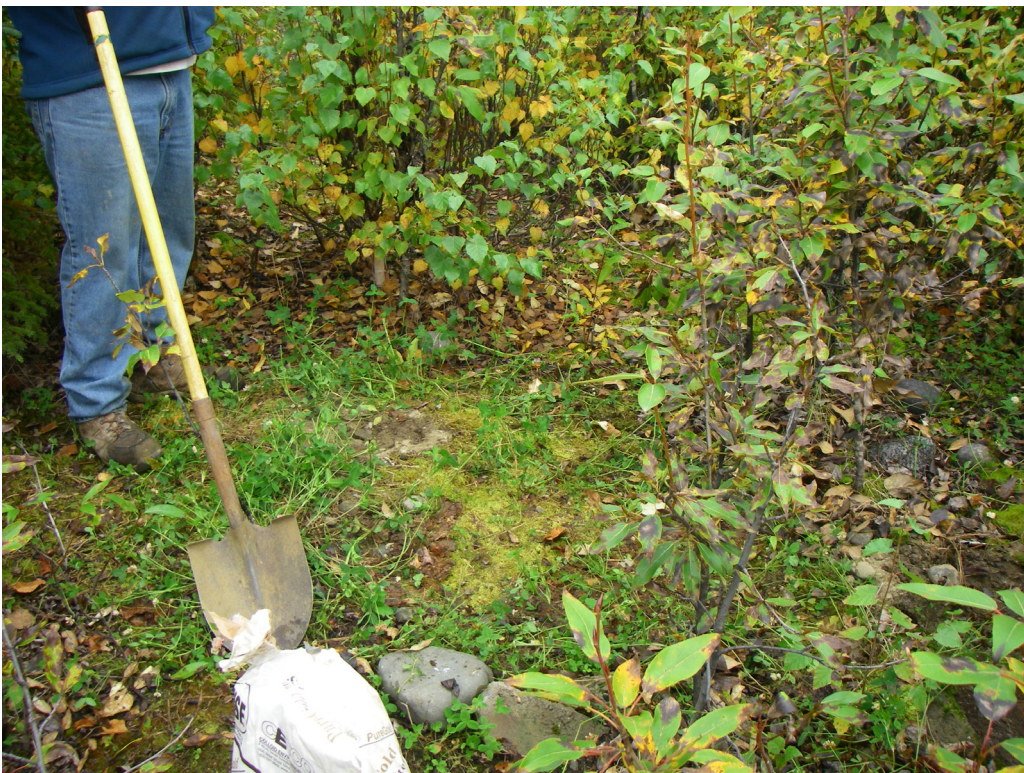
Photograph 6: B-11MW decommissioning completed.
