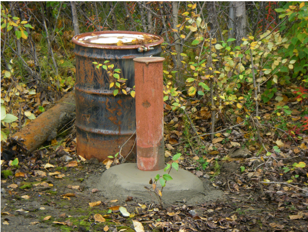
Photograph 8: GW-2 after rehabilitation completed.
