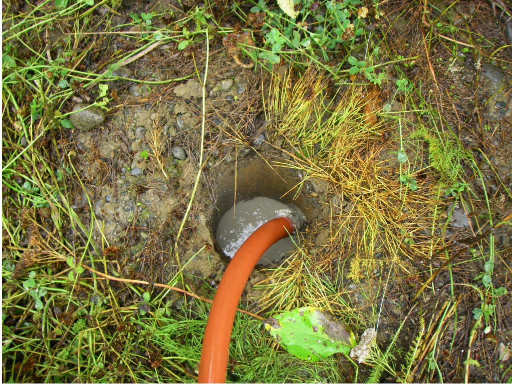
Photograph 3: Pumping volclay into GW-1.
