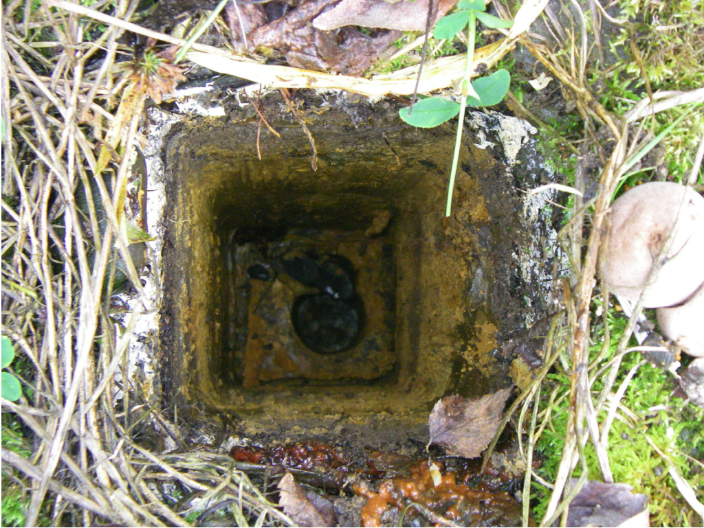
Photograph 5: Remaining hole in B-11MW after with casing removal..
