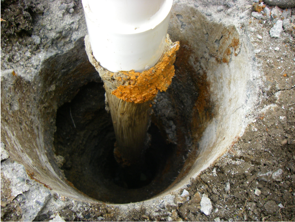
Photograph 7: GW-2 with old monument removed and new casing extension attached.
