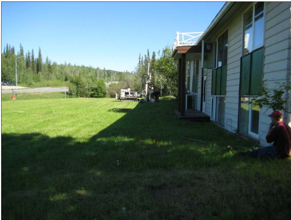
Photo 02 - Looking north along west side of structure at installation of SB-15
