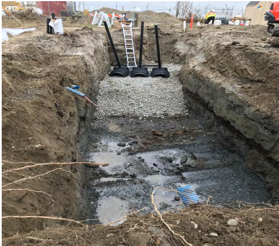
Photo #6 – Start of Installation of Infiltrators™ with Sewer Rock.
