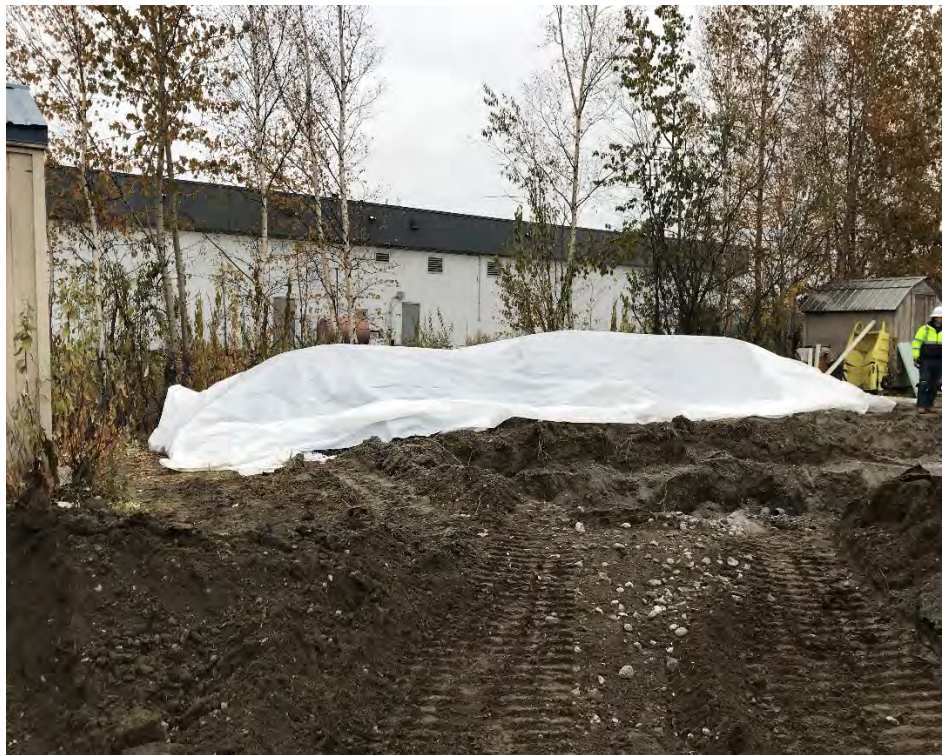
Photo #8 - Covered 40 CY Stockpile of Contaminated Soil (looking north)
