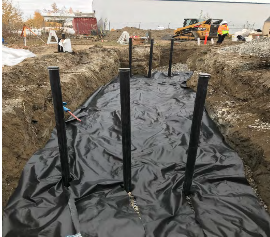
Photo #9 – Installation of Fabric Material of Completed Infiltrator Drainfield (looking east).
