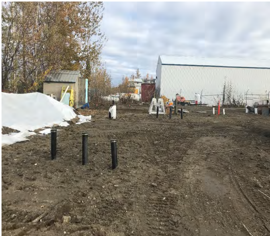
Photo #10 – Completed Installation of Backfill over 2021 Drainfield with Observation Pipes
