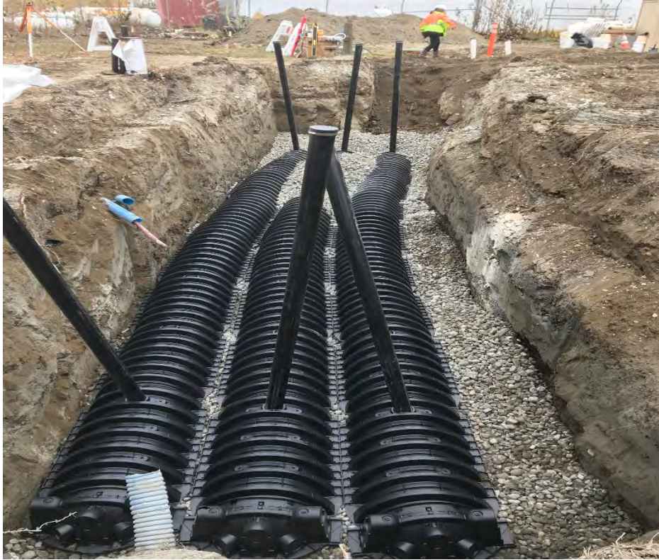
Photo #7 - Completed Installation of Infiltrators prior to placement of Fabric Material
