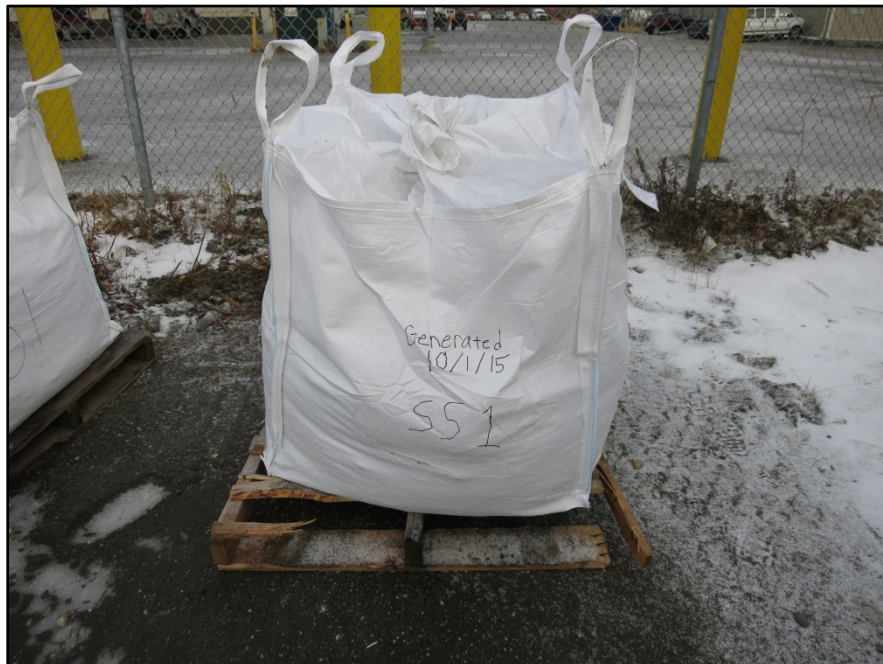
Photograph 10: All cuttings generated during drilling were containerized in a super sack and staged as pictured here. (Oct 1, 2015).
