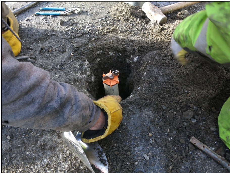
Photograph 8: Repairing the surface vault at MW-2. (Oct 1, 2015).
