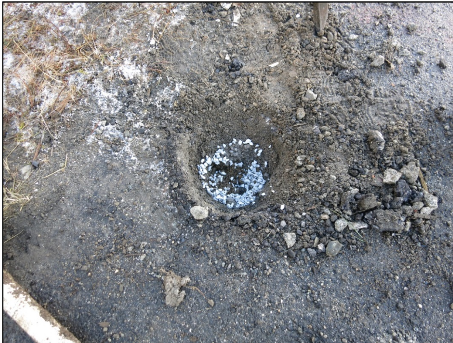
Photograph 2: Decommissioned well MW-3. Bentonite is visible in photo. Clean gravel was filled over bentonite to match surface grade. (Sep 30, 2015).
