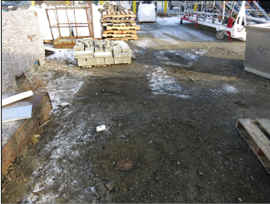
Photograph 7: Completed monitoring well MW-1R with flush mounted vault. Photo faces north. (Oct 1, 2015).
