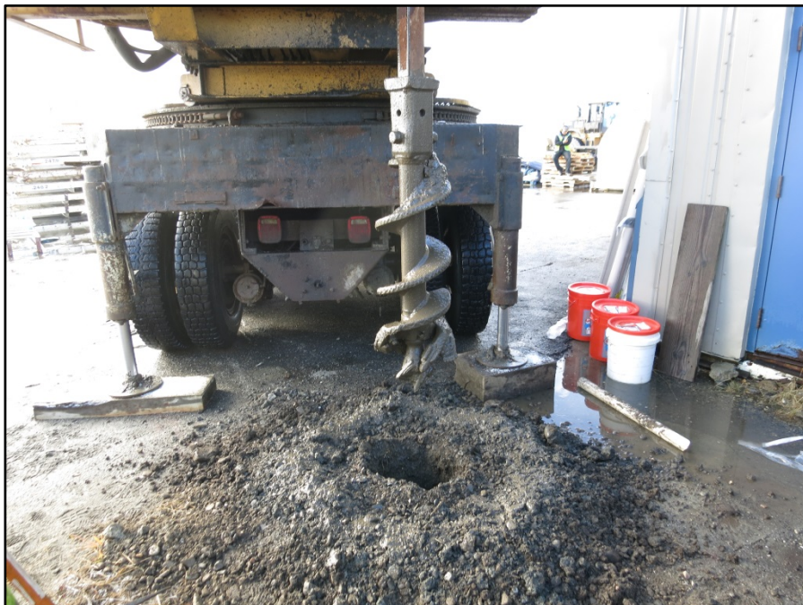
Photograph 4: Larger truck-mounted auger drill rig at MW-3R. (Sep 30, 2015).
