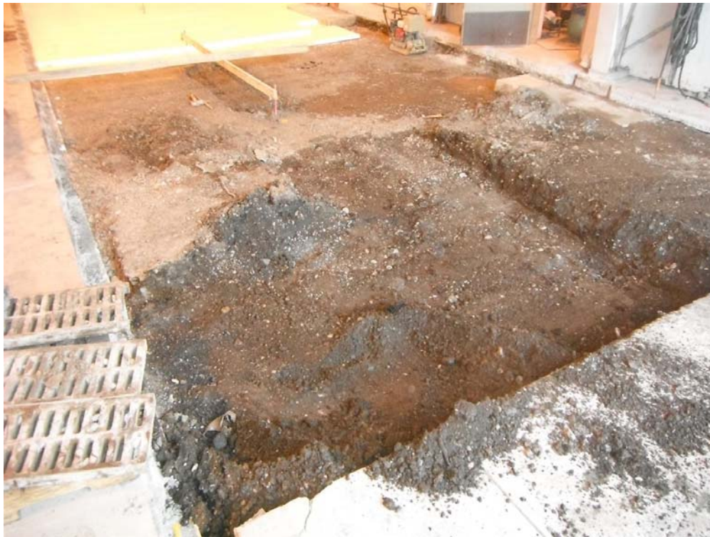
Photo 3: Excavation Area A – Initial soil removal.
