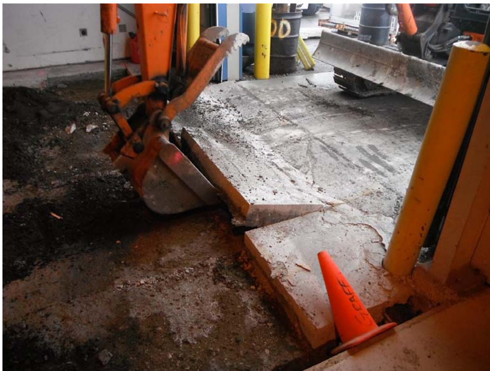
Photo 4: Excavation Area A – Remaining concrete section removal.
