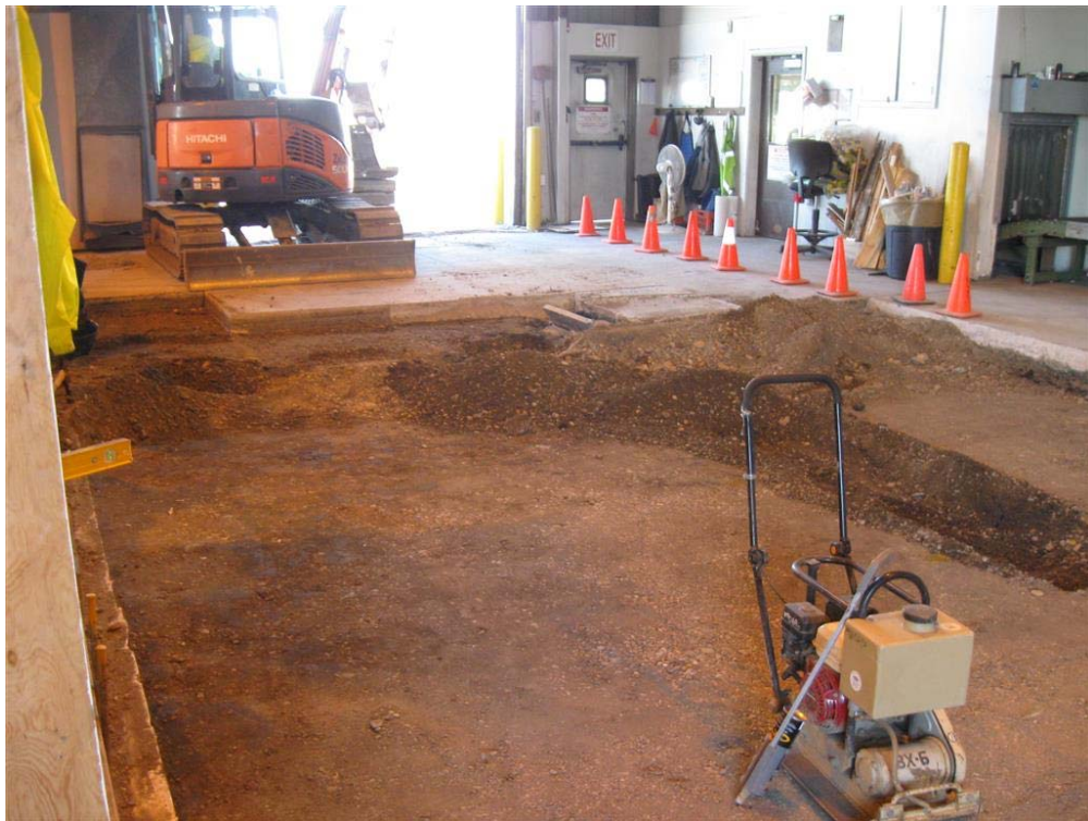
Photo 6: Excavation Area B – Exposed area with fuel hydrocarbon odor.
