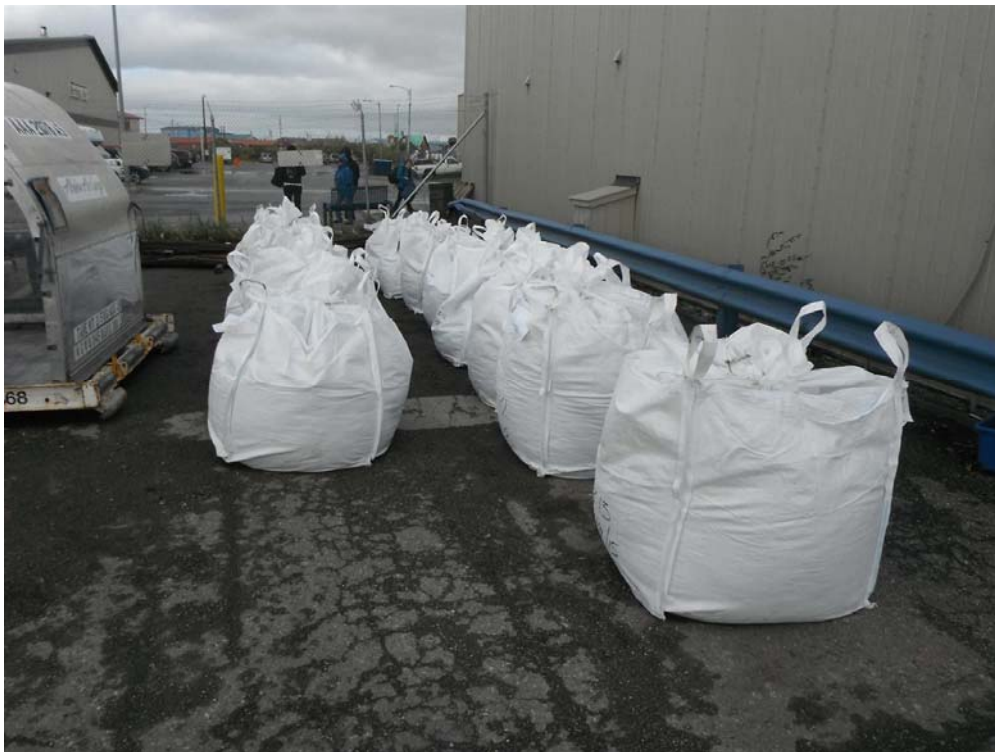
Photo 10: Excavated soil contained in lined super-sacks.
