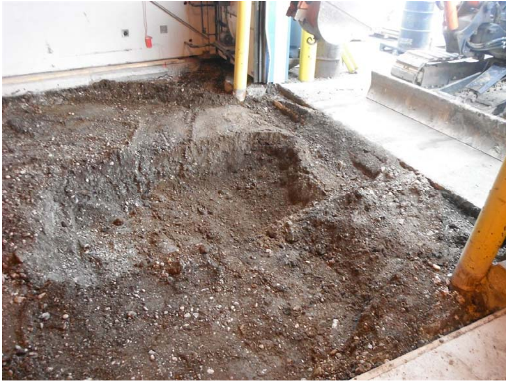
Photo 5: Excavation Area A – Excavation for drainage sump.
