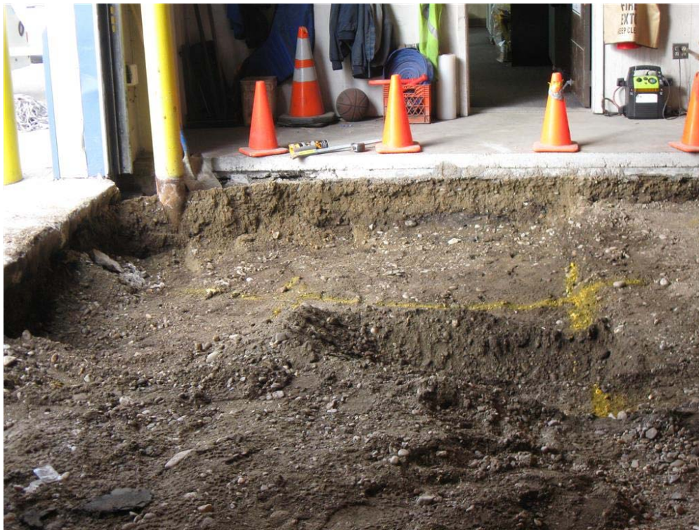
Photo 8: Excavation Area B – Excavation for drainage sump.
