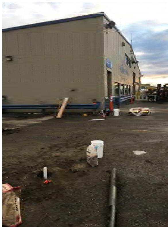
Photo 4: Installing monitoring well casing at replacement well MW-1R2. 10/5/2016
