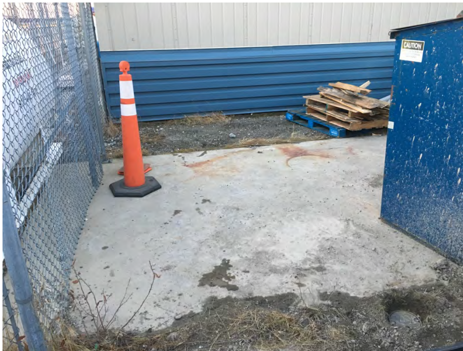
Photo 6: Monitoring well MW-5 site after installation. Well is installed in gravel between asphalt of the parking area and cement pad next to dumpster. 10/7/2016
