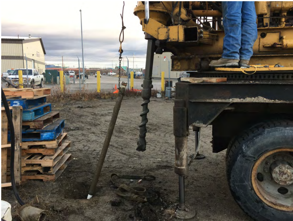
Photo 1: Decommissioning monitoring well MW-1R using drill rig and winch line. 10/5/2016
