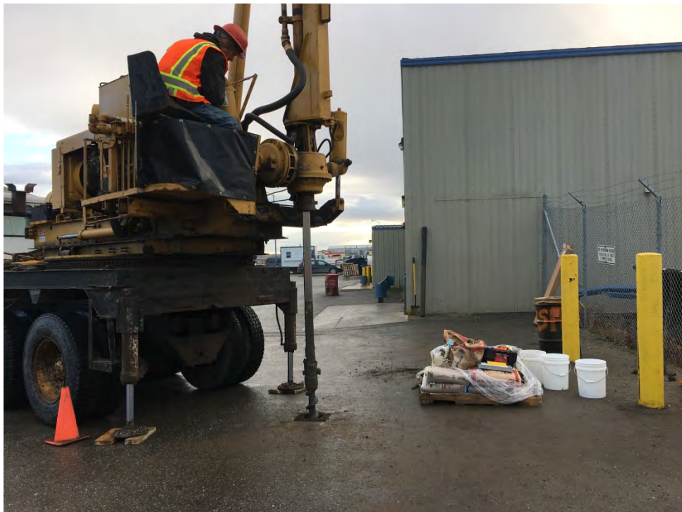
Photo 2: Drilling boring for monitoring well MW-4. 10/5/2016
