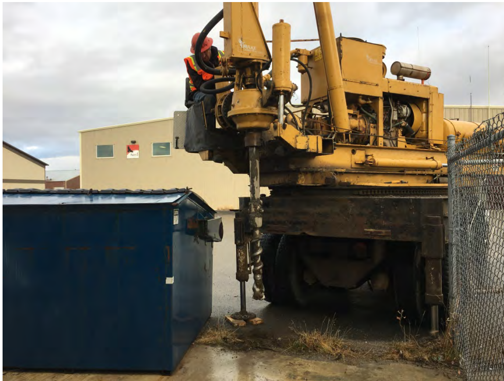
Photo 3: Drilling boring for monitoring well MW-5. 10/5/2016
